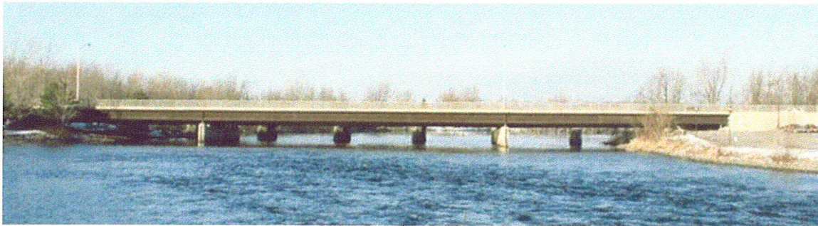
Fig. 1.1. RT11 bridge over Raquette river in Potsdam, NY.
