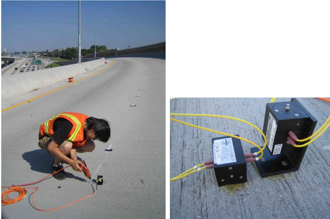
Figure 23 Installation of Fiber Optic Accelerometer
