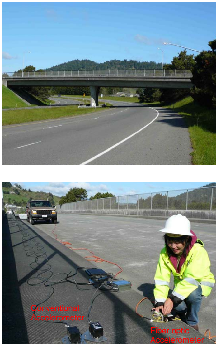
Figure 19 Test at Painter St. Overcrossing
