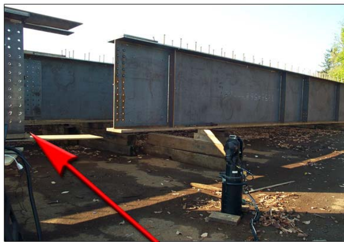
Measuring Splice Plate Hole Locations
