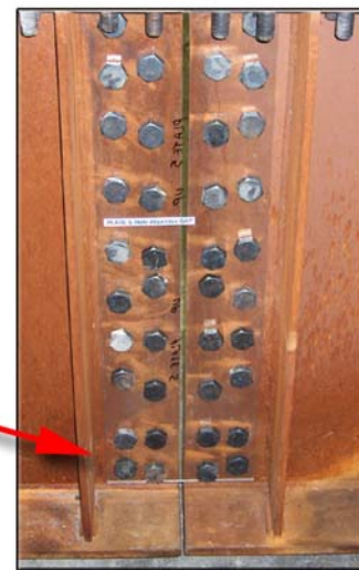
FIGURE 12 Custom splice plates designed from laser system measurements.
