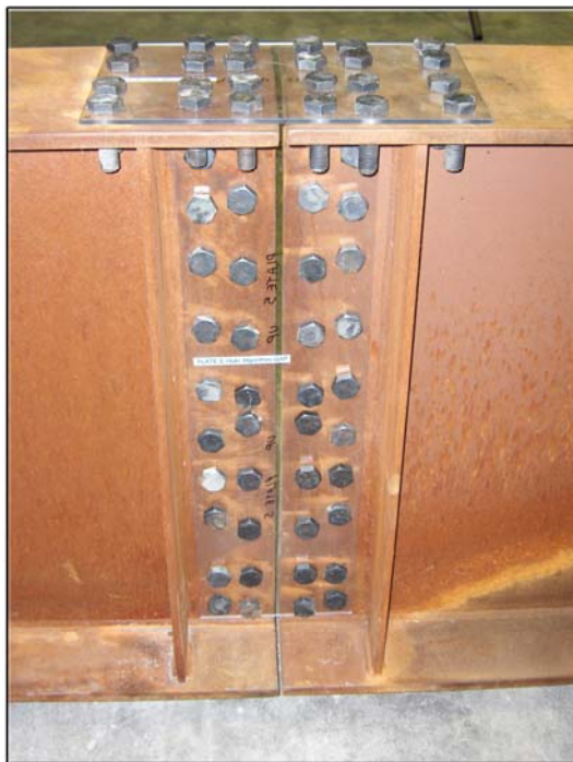
FIGURE 11 Virtual fit-up of girders for splice plate design.
