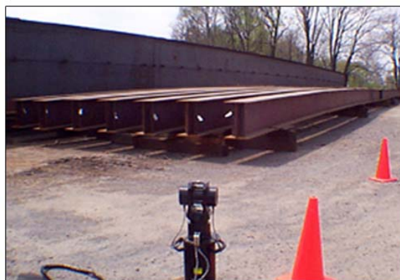
Measuring Blocked Position of Girder in Assembly Yard
