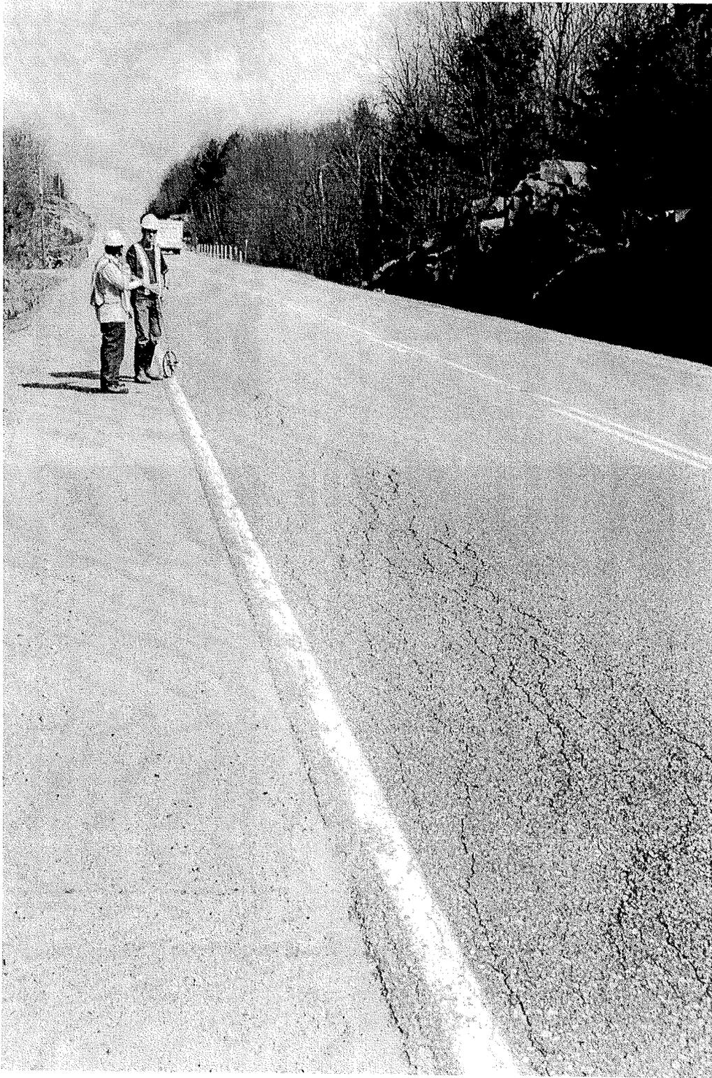
: Figure 4.43 Illustrative picture for longitudinal cracking in section 118-5.
