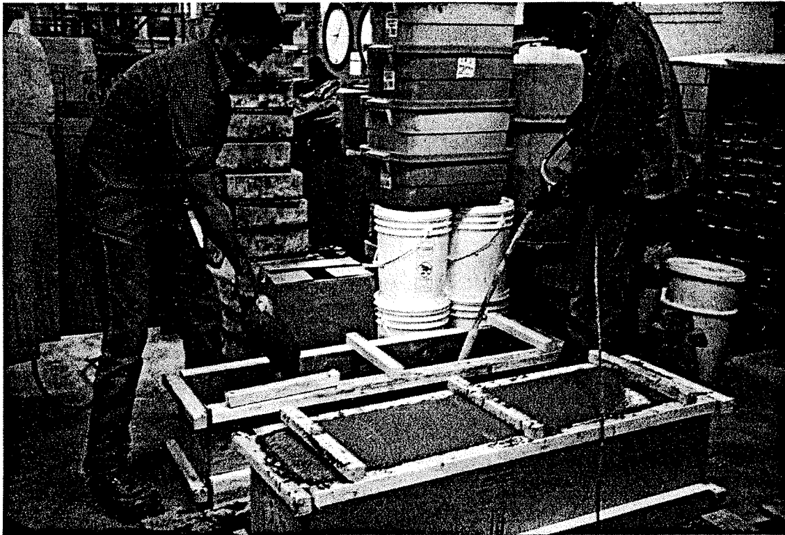
Photo 6 Casting of Basalt Reinforced Concrete Beams
