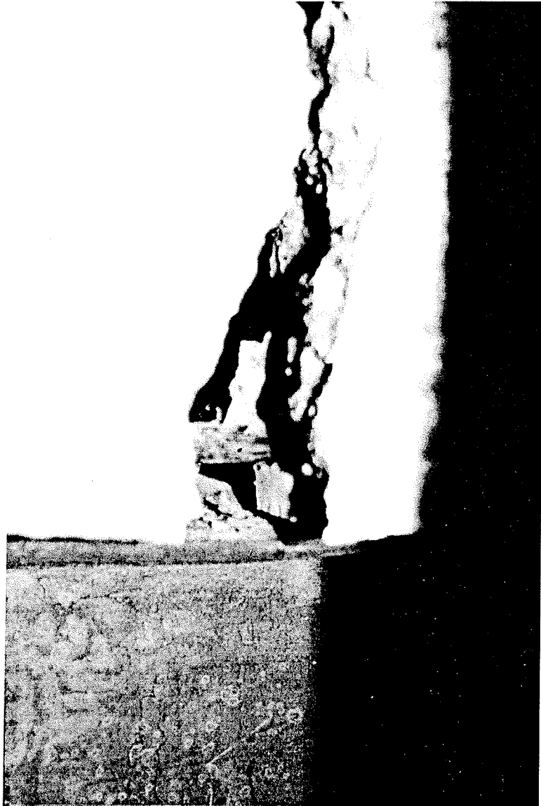
Photo 12 Close-up showing maximum width of crack Maximum crack width = 50mm(2 in.)
