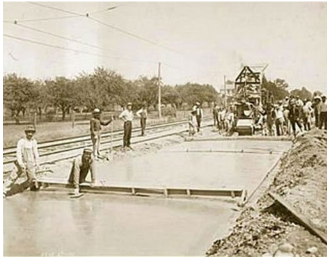
FIGURE 1. Paving Woodward Avenue in 1909 (Michigan in Pictures)
