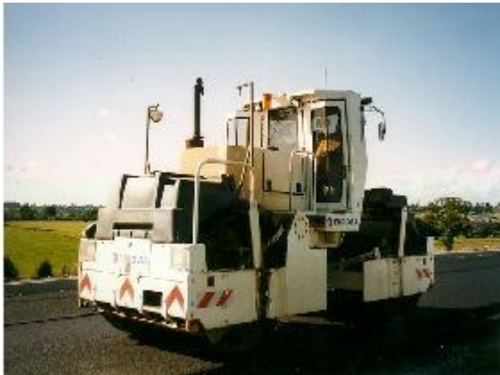
Figure 10 The compactor used for the full-scale trials.
