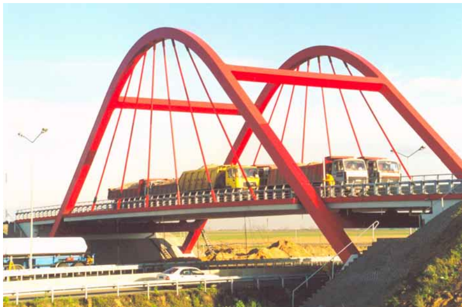
FIGURE 4 Arch viaduct A016 over highway A4 during load tests.
