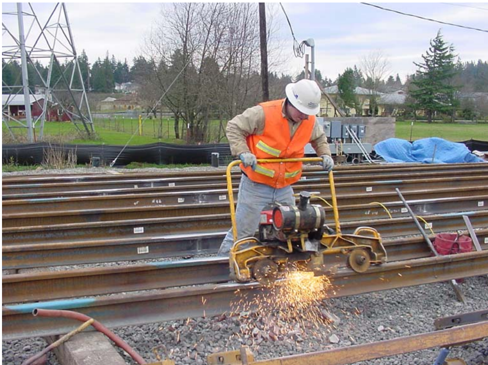
FIGURE 6 Interstate MAX light rail construction worker grinding string with profile grinder at Ruby Junction Maintenance Facility Expansion Project.
