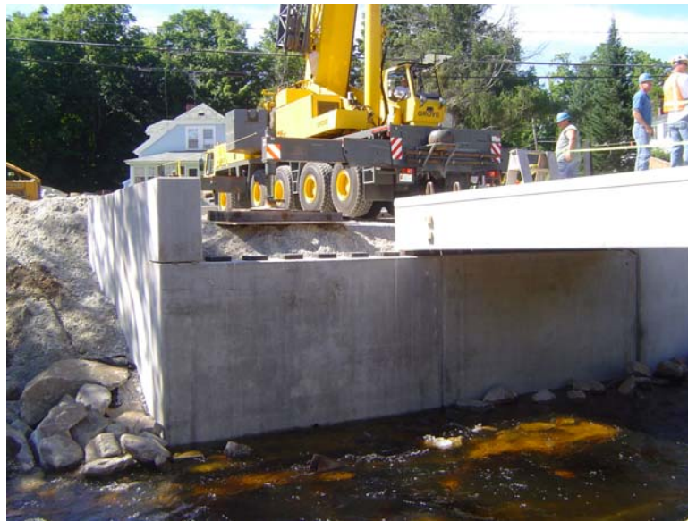
FIGURE 12 Rapid bridge replacement.
