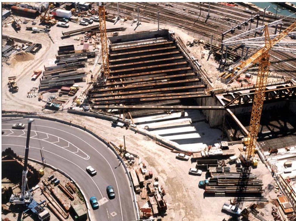
FIGURE 4 Central Artery Tunnel jacking pit.
