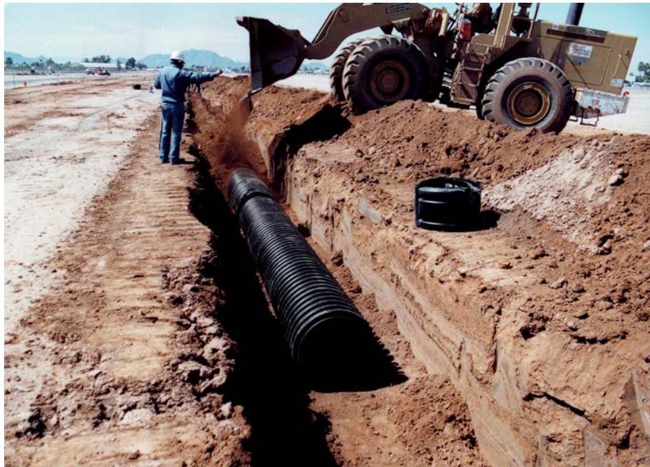
FIGURE 3 Corrugated PE installation.
