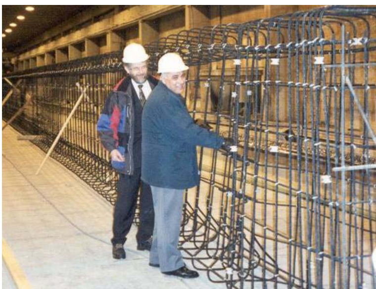
FIGURE 2 CFRP stirrups for prestressed girders.
