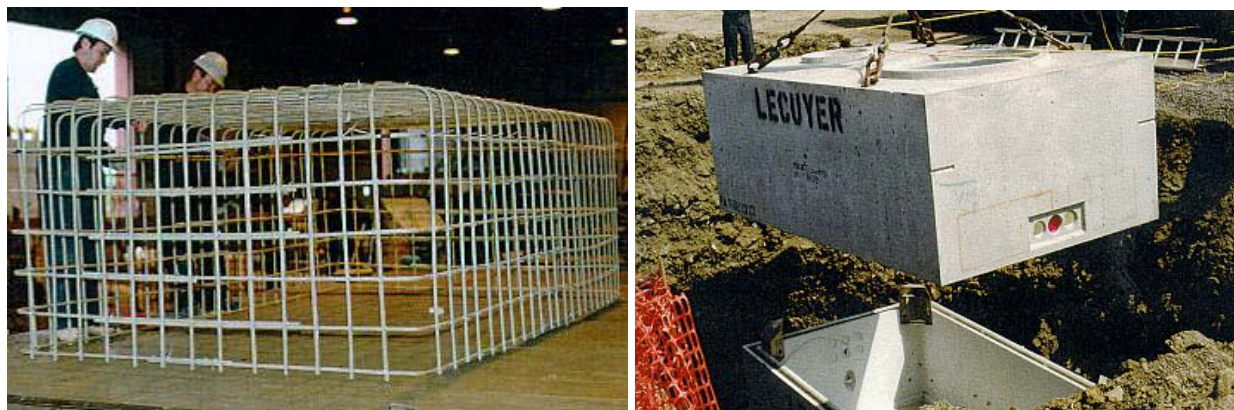
FIGURE 3 GFRP reinforced underground precast concrete chambers.
