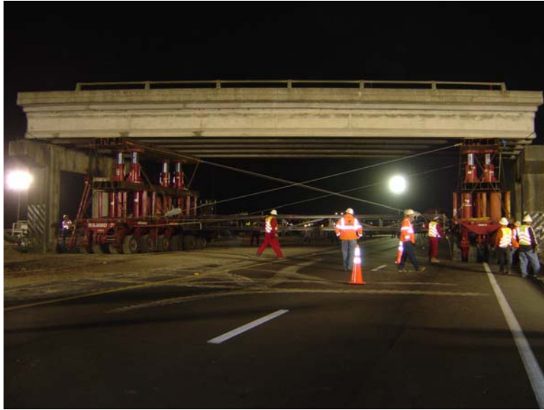
FIGURE 11 Complete bridge change-out.
