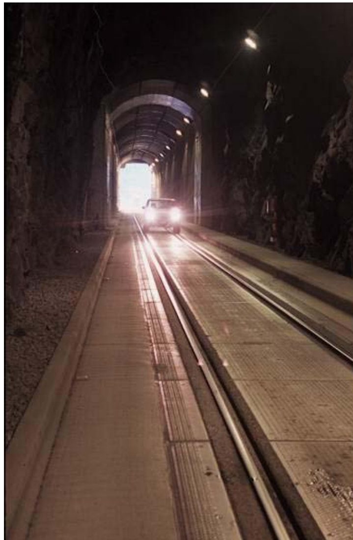
FIGURE 5 Composite roadway and rails in Whittier Tunnel.
