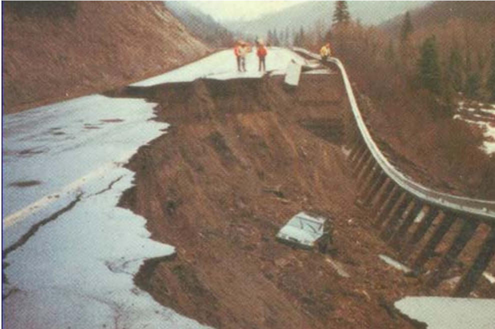
FIGURE 1 Recurring landslide on Colorado State Highway 133 at McClure Pass, west of Aspen, in spring 1993—a good reason for research.
