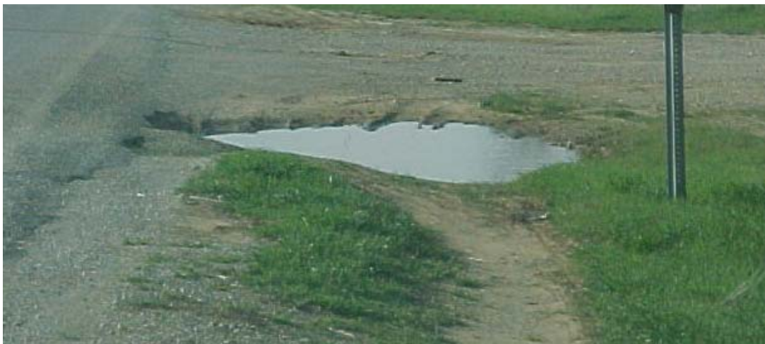
FIGURE 15 Water standing where no turnout is installed.
