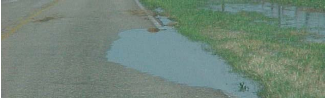
FIGURE 1 Inadequate ditch forces water onto the pavement.
