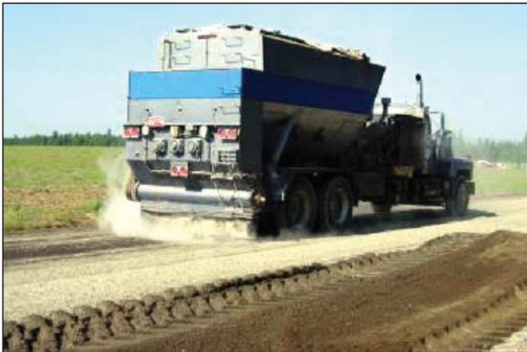
FIGURE 4 Placing cement dry.
