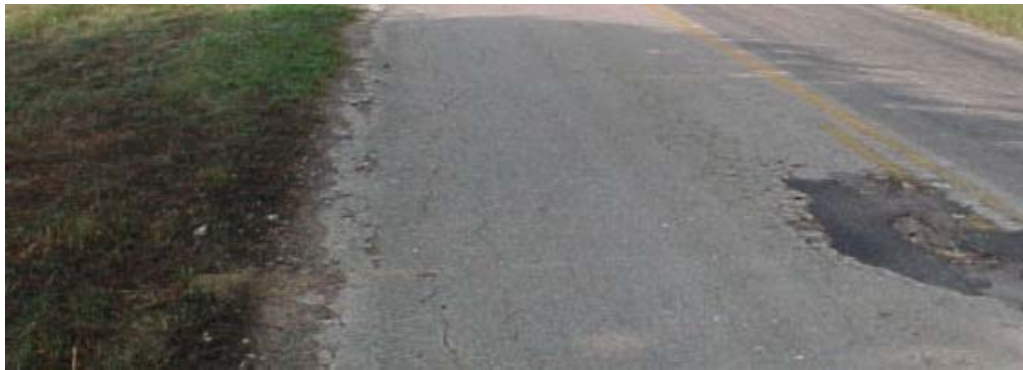
FIGURE 3 Narrow pavement creates edge problems.
