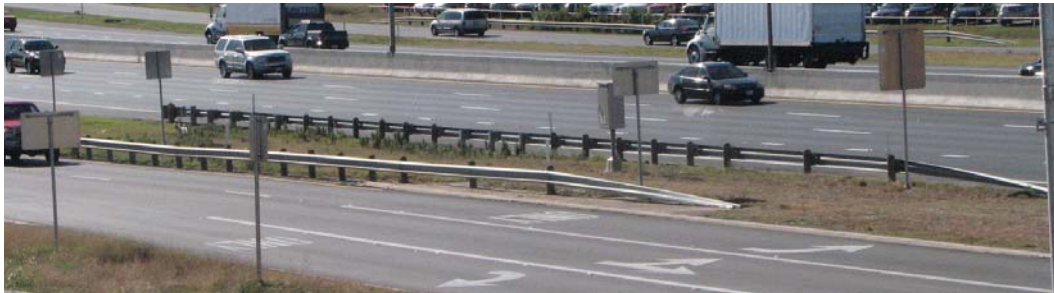
FIGURE 9 Guardrail (350 ft) installed to protect cabinet; move cabinet instead.
