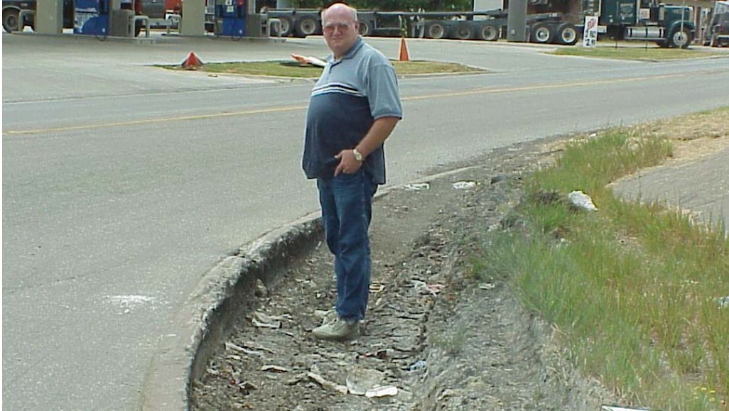
FIGURE 2 Truck traffic has created a severe rut along pavement, even behind curb.
