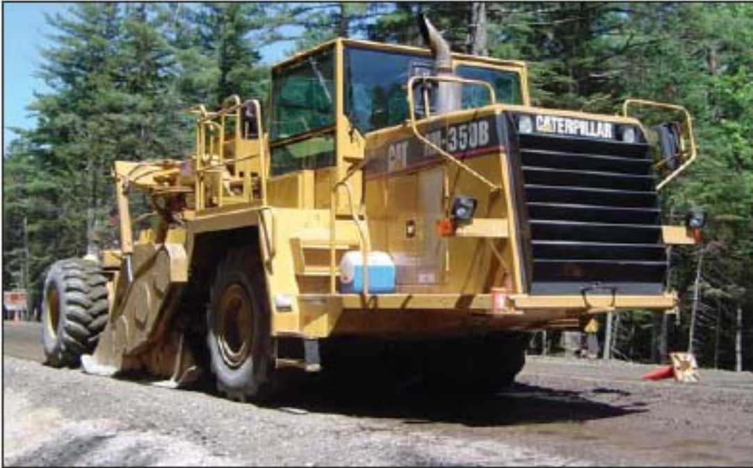
FIGURE 3 Pulverizing a failed asphalt pavement.
