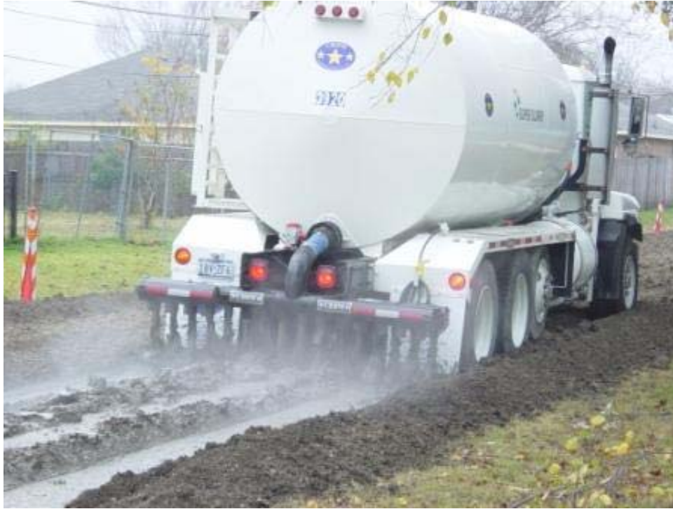
FIGURE 5 Placing cement in slurry form.
