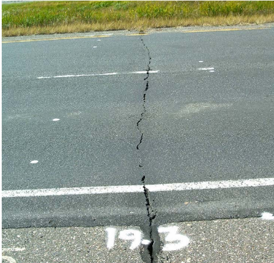
FIGURE 2 Reflected transverse crack through the slurry seal .
