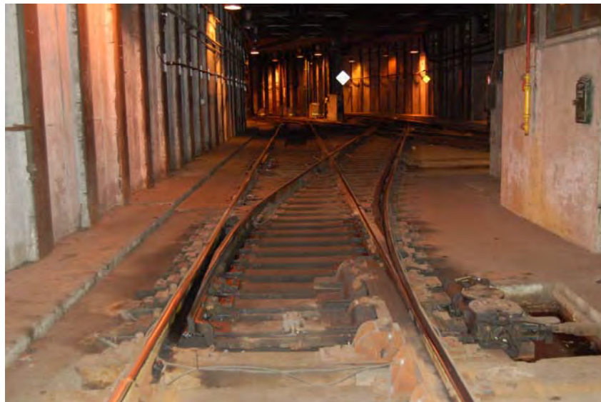
FIGURE 7 Fully guarded switch.
