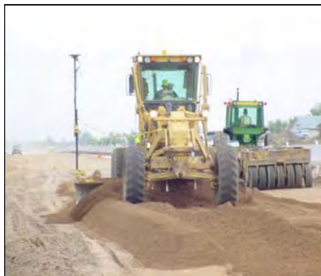
FIGURE 1 Automated machine guidance.
