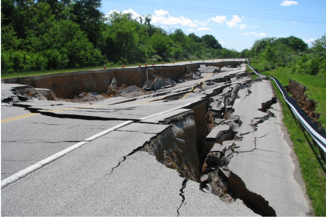
FIGURE 3 SR-7 in Maury County, Tennessee, after intense rainfall and record-level flooding in May 2010.
