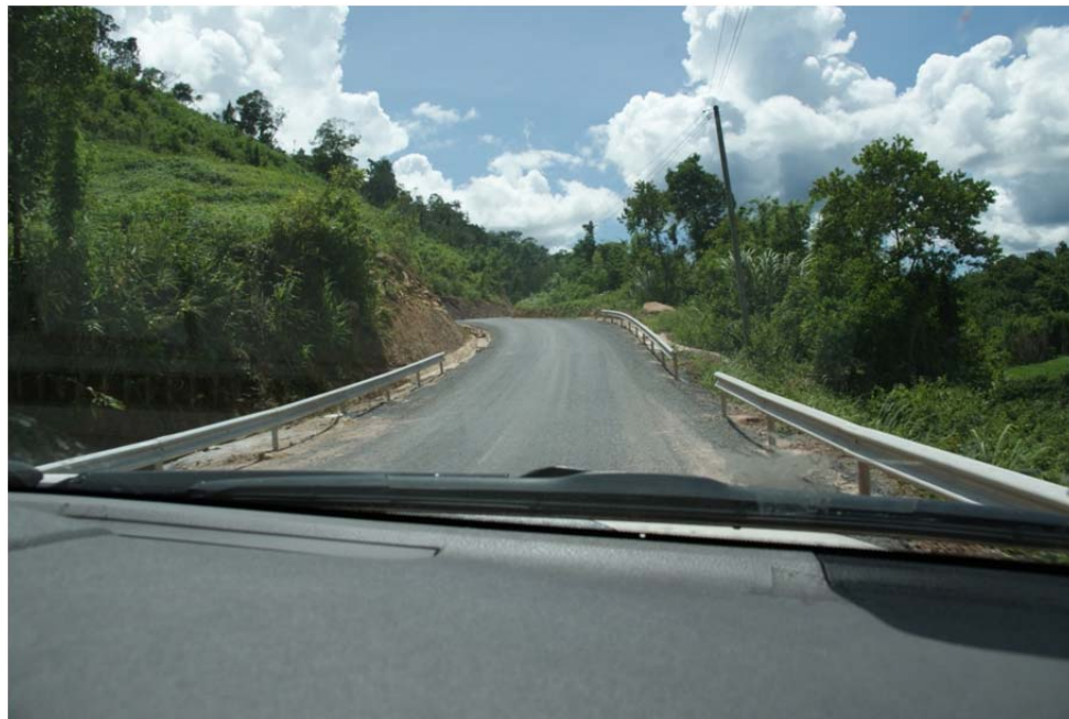
FIGURE 2 Example of discontinuous, open W beam steel barrier with no end treatments.
