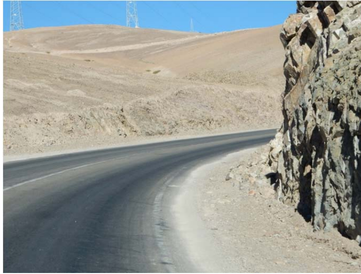
FIGURE 6 Curved zone: poor side delineation, unprotected obstacle and minimal sight distance
