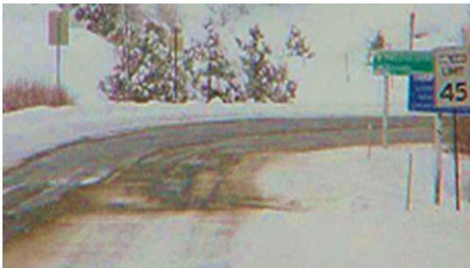
FIGURE 4 Extra material applied at hazardous curve.
