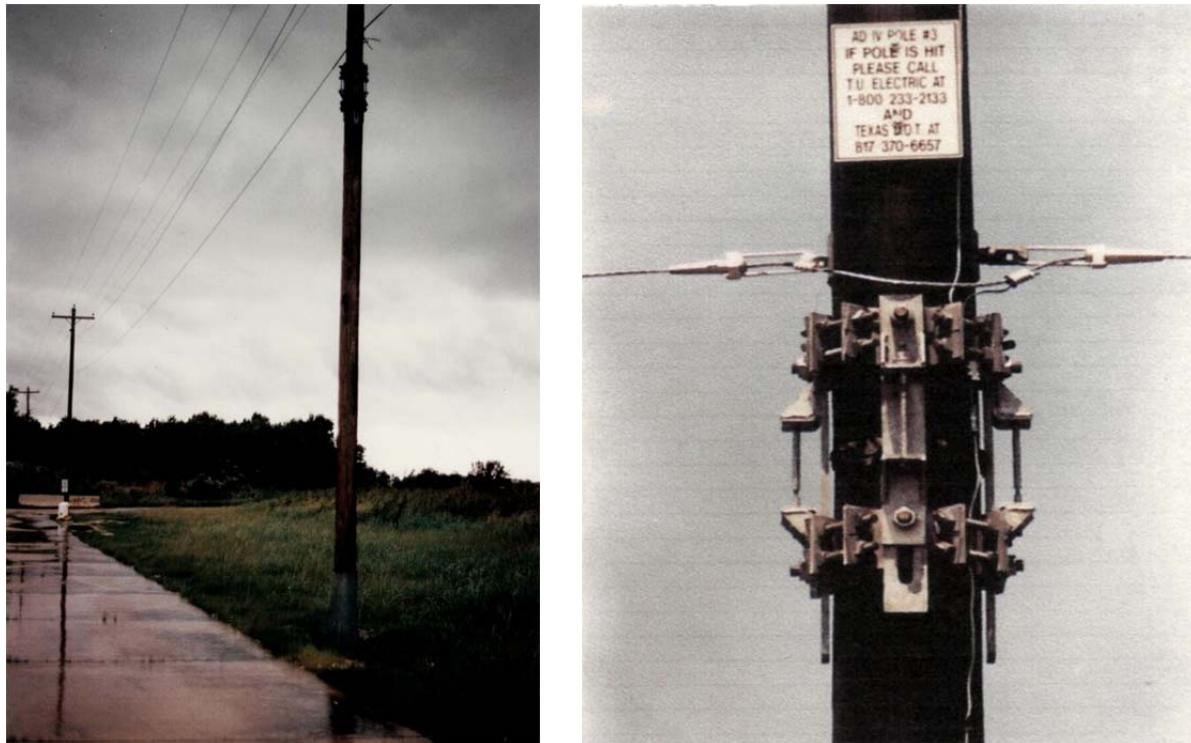
FIGURE 5 Steel reinforced safety pole (SRS pole).
