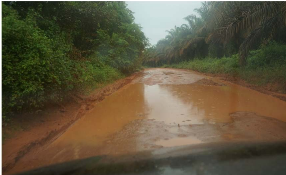
FIGURE 8 Road where water is not drained either across (by use of a pipe culvert) or away from the roadside, but is left to pool on the road surface. Vehicle traffic will destroy the road at this location.
