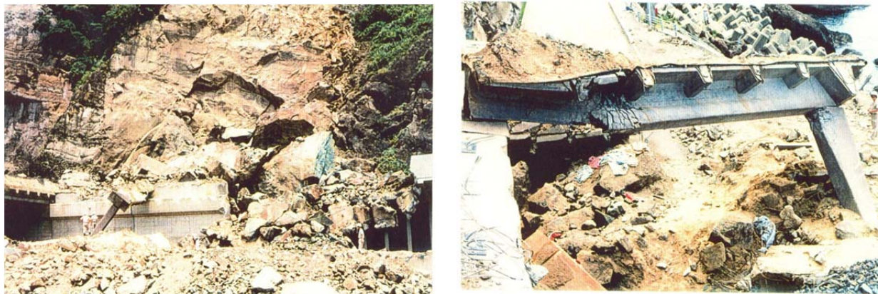
FIGURE 1 Failure of rock-shed caused by falling rock in Etizen, Japan, July 1989 (Masuya, 1997).
