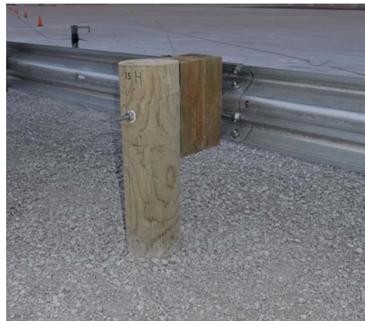
FIGURE 3 Arizona G4(2W) guardrail system with round PP posts.
