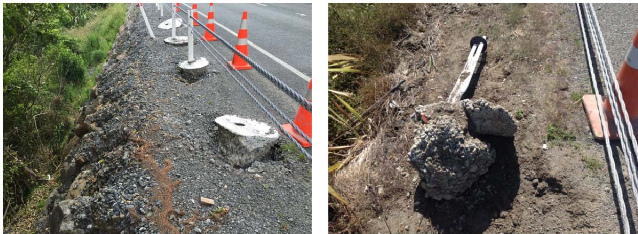
FIGURE 2 Post failures (21).
