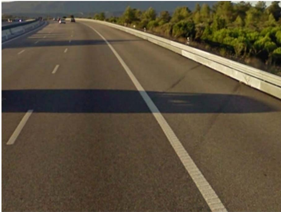
FIGURE 3 Google Street View image with carriageway departure skid marks and evidence of restraint system substitution
