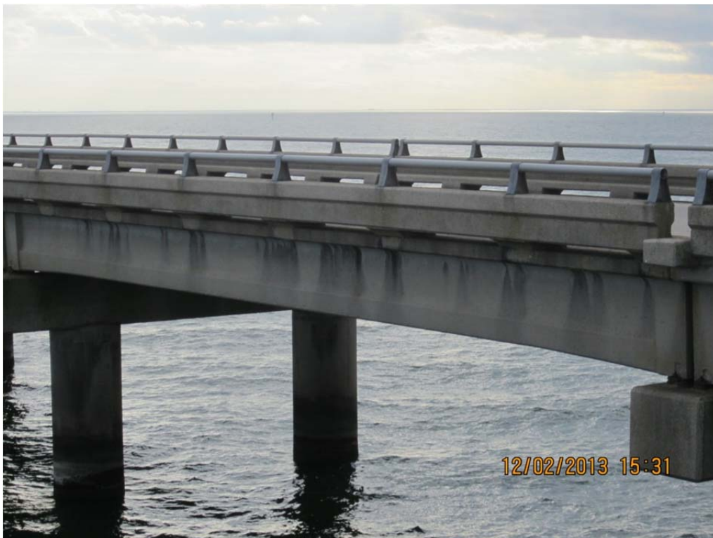
FIGURE 2 Photo of southbound causeway bridge rail.
