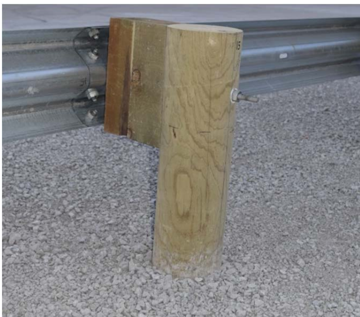
FIGURE 3 Arizona G4(2W) guardrail system with round PP posts.
