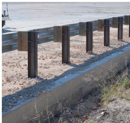
FIGURE 8 Details and photos of (a) side-mounted and (b) top-mounted guardrail systems attached to culverts.
