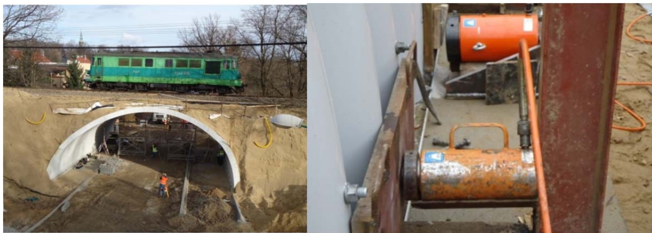
FIGURE 17 Mechanically tensioned arch construction in Poland showing the jacks used.
