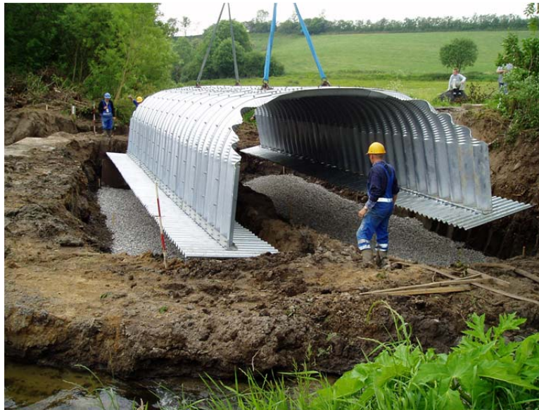
FIGURE 14 Steel arch structure with corrugated steel footers being installed.
