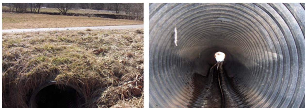
FIGURE 1 Ohio DOT installation of 24-in. (600-mm) diameter culvert after 27 years in mine acid run-off.
