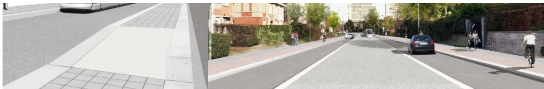
FIGURE 6 Articulation using similar contrasting kerbs for tram lane and platform edges.
