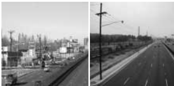
FIGURE 2 Route 30, Camden—Admiral Wilson Boulevard.
