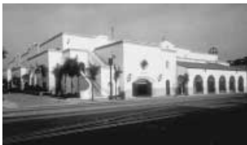
FIGURE 5 Parking garage, Santa Barbara, California.
