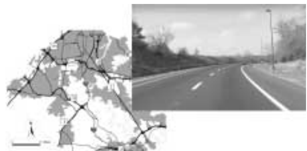
FIGURE 18 I-97 (I-695 to US-50), Anne Arundel County, Maryland.
