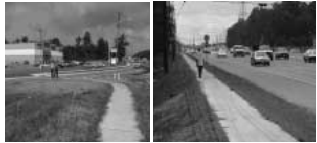
FIGURE 6 Route 1, North Brunswick.
