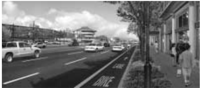
FIGURE 15 Improved suburban highway.
