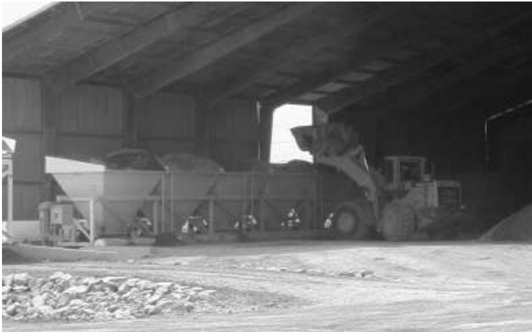
FIGURE 1 Covered aggregate stockpiles and cold feed bins.
