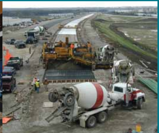
Slip form paving to extend Illinois North-South Tollway (I-355)
