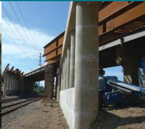
Railway overpass of advanced, weldable, weathering steel, Lake Villa, Illinois
