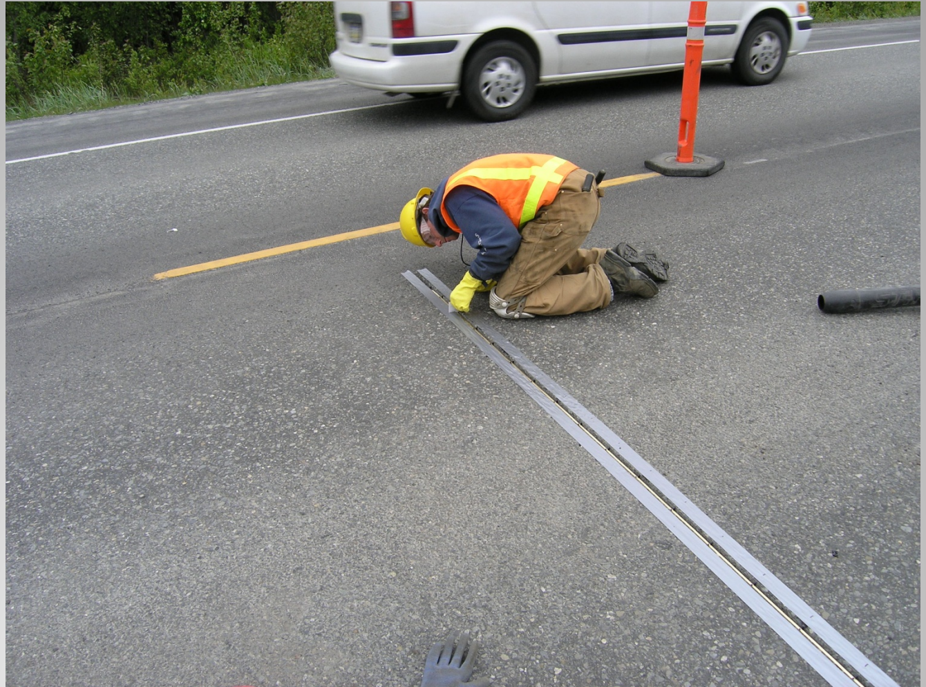
Piezo Installation - Placement
