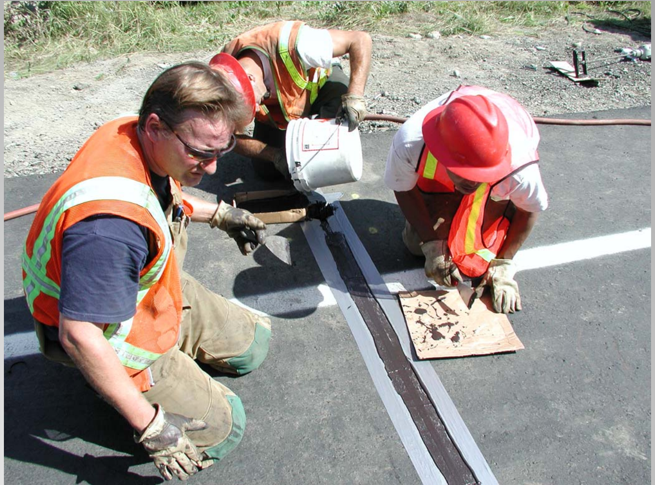
Piezo Installation - Epoxy
