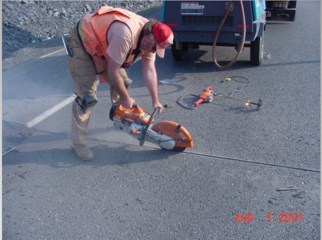
Piezo Installation - Saw Cut
