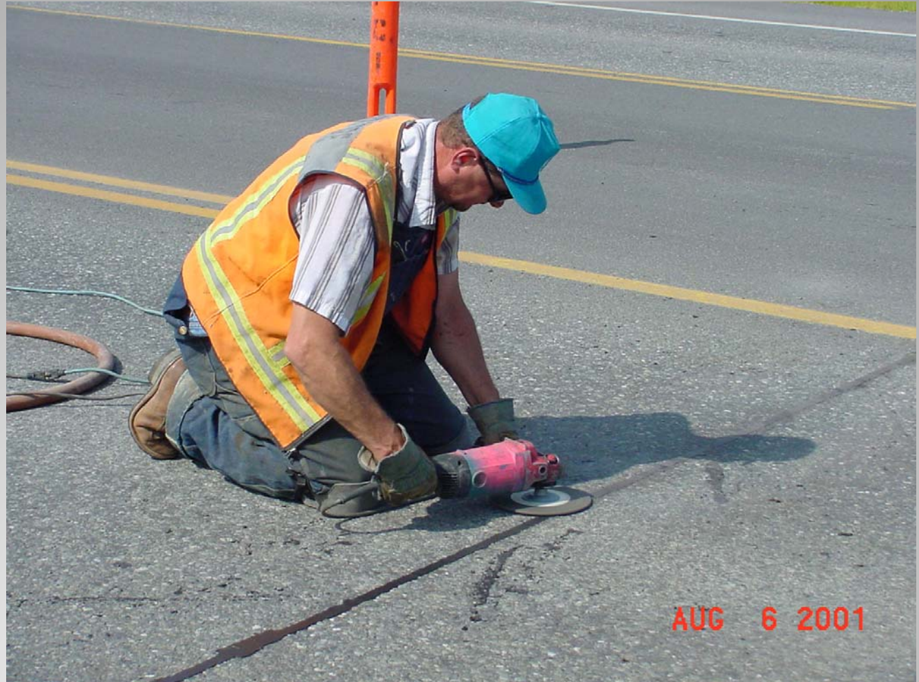
Piezo Installation - Grind
