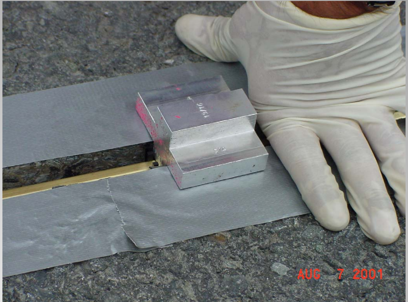
Piezo Installation - Placement
