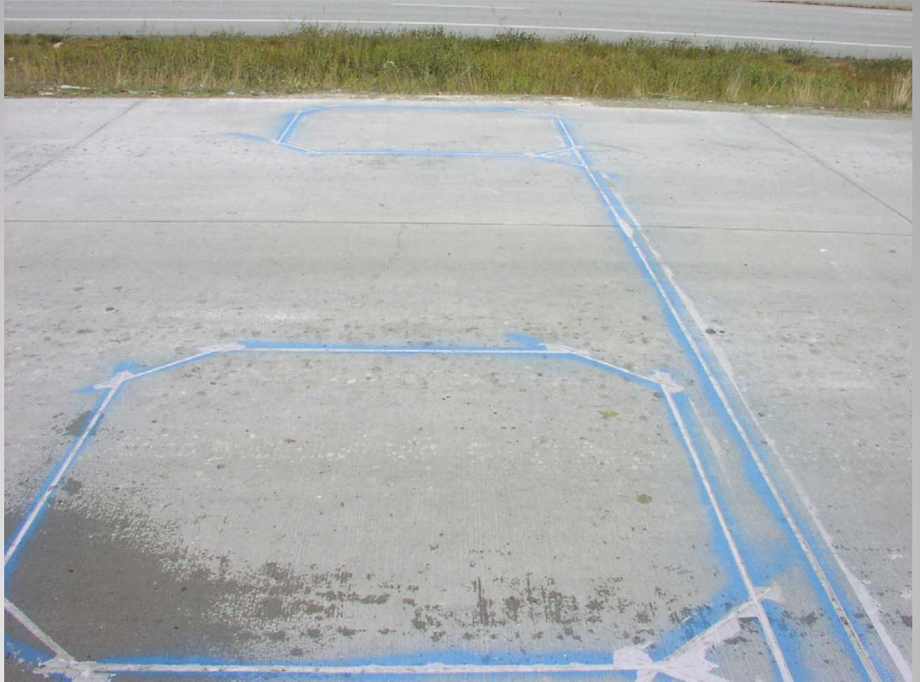
Saw Cut Loops
