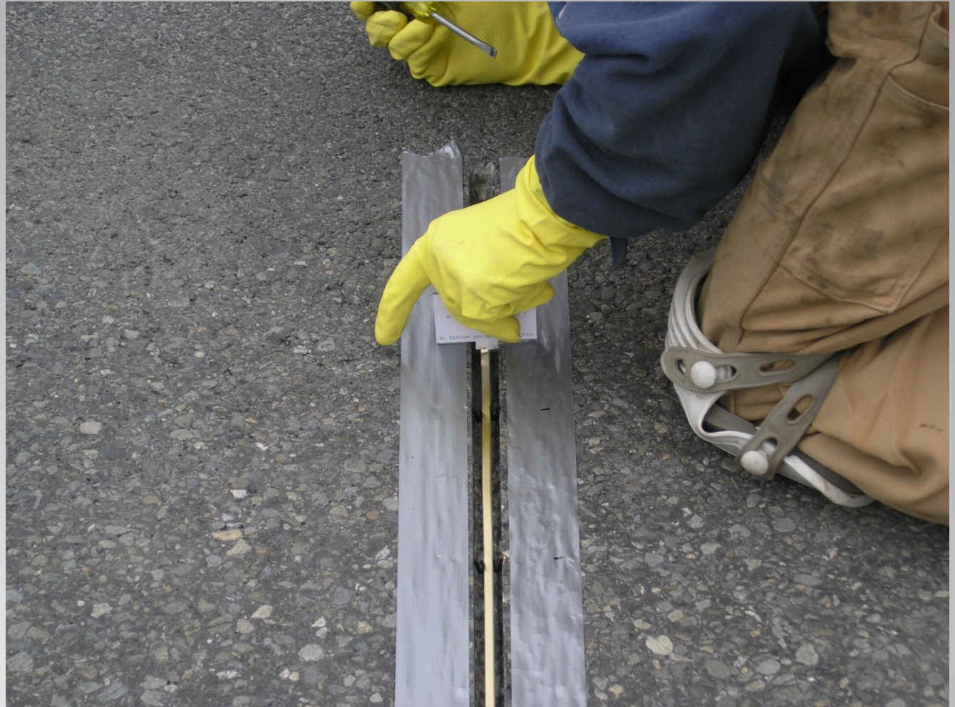
Piezo Installation - Placement
