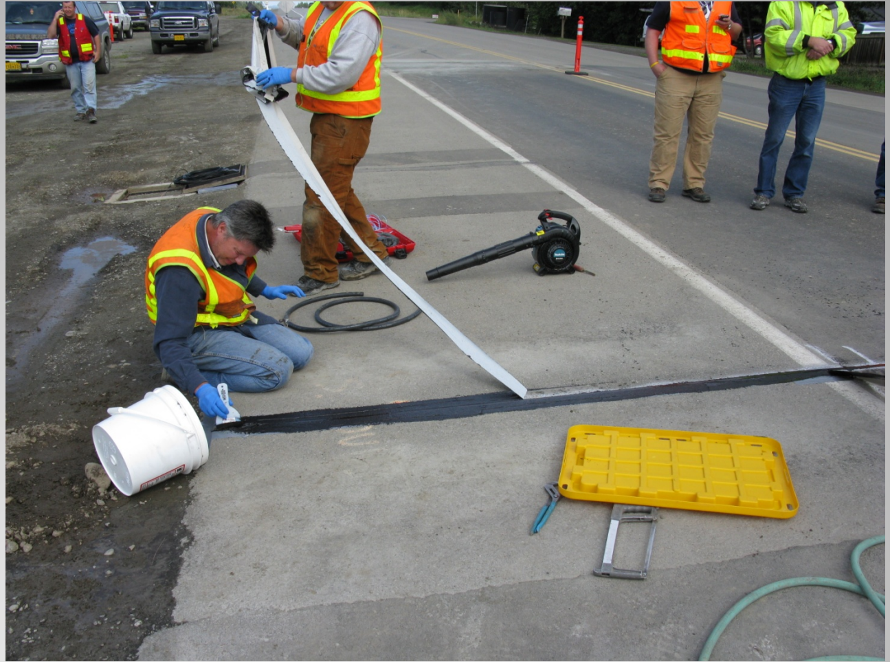
Piezo Installation - Clean up
