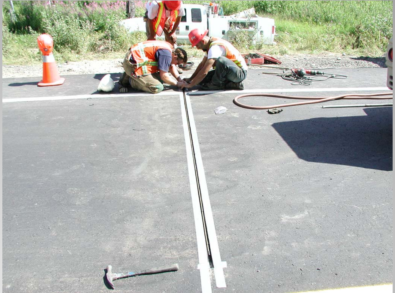
Piezo Installation - Placement
