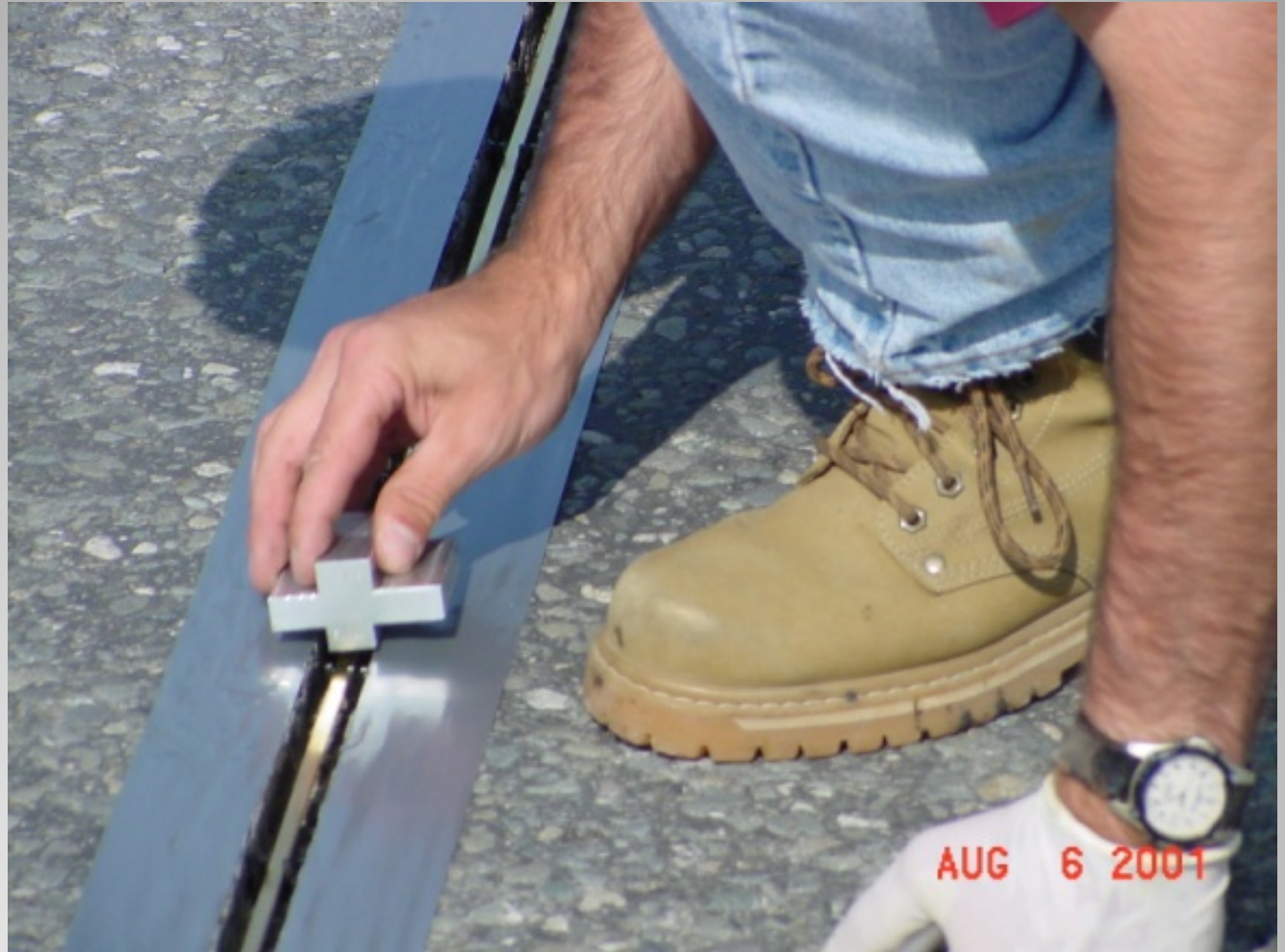
Piezo Installation - Placement
