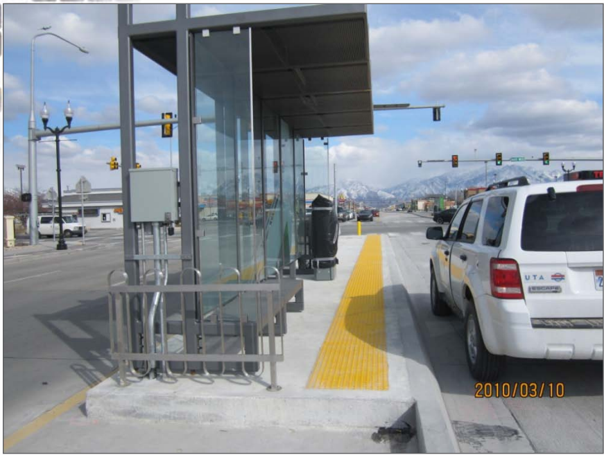
Center running canopy
