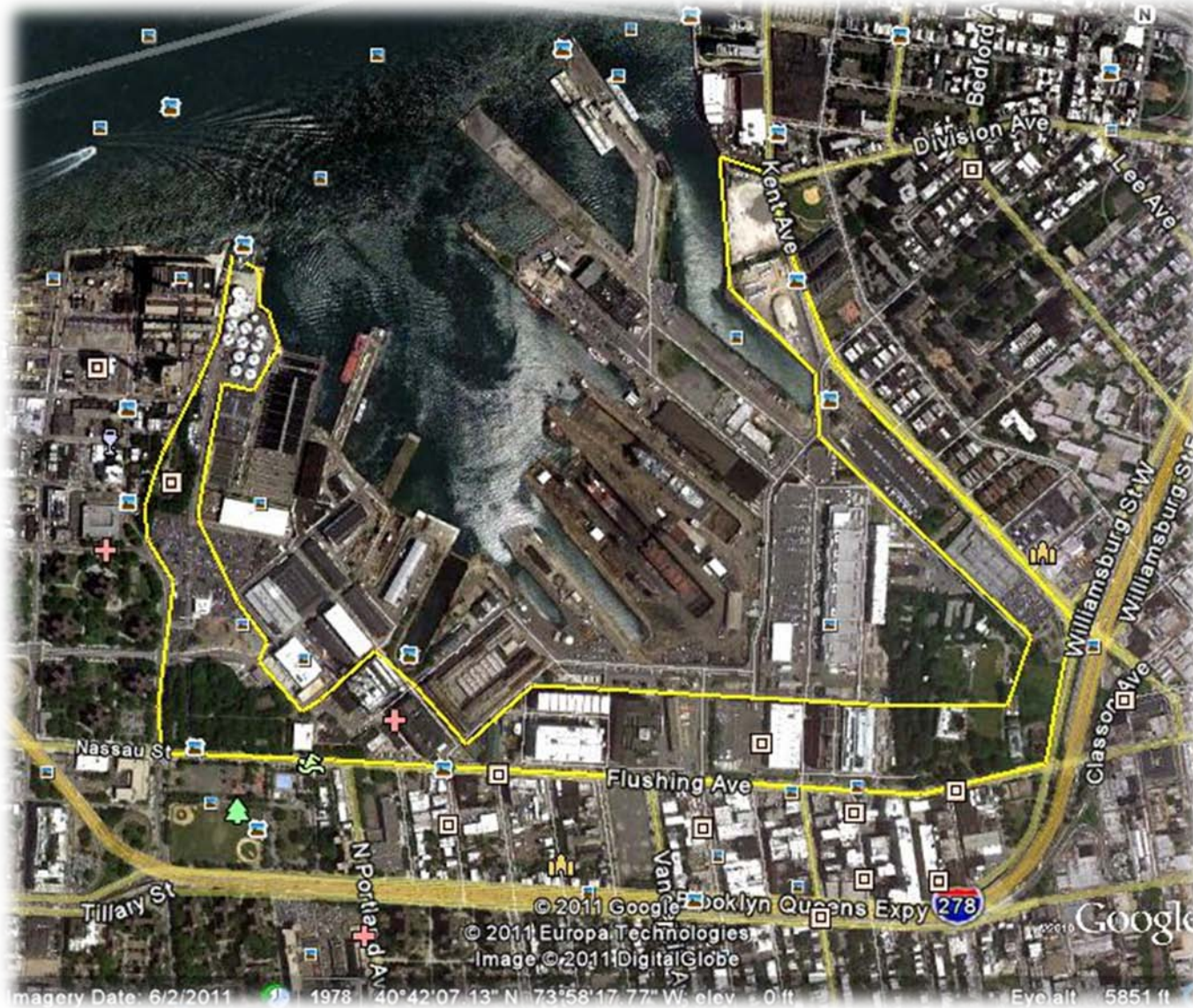
Brooklyn Navy Yard – 6 Graving Docks – 3 Inactive
