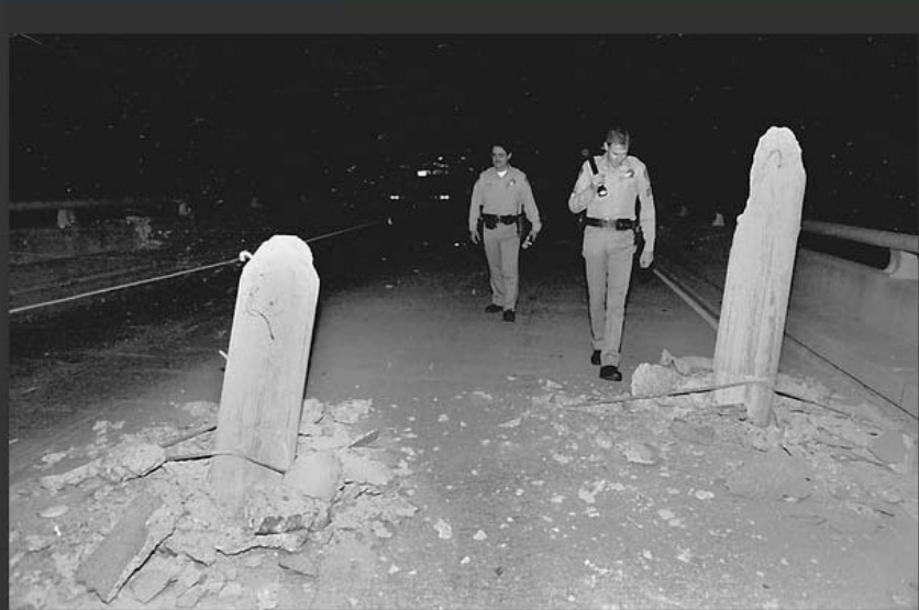
Highway Patrol officers check out the Harkins Slough Bridge on Highway 1 where bridge supports pierce the shaken and fallen elevated highway hours after the quake. Dan Coyro/Sentinel
