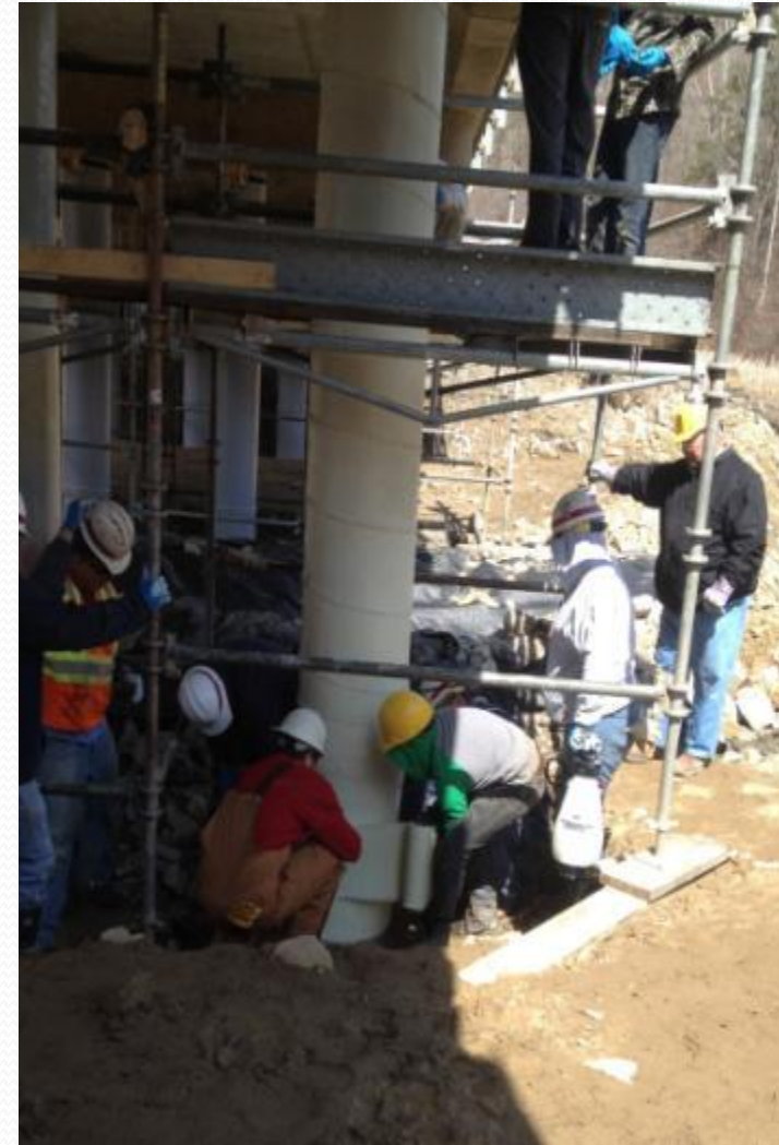
Wrapping the piles with FRP
