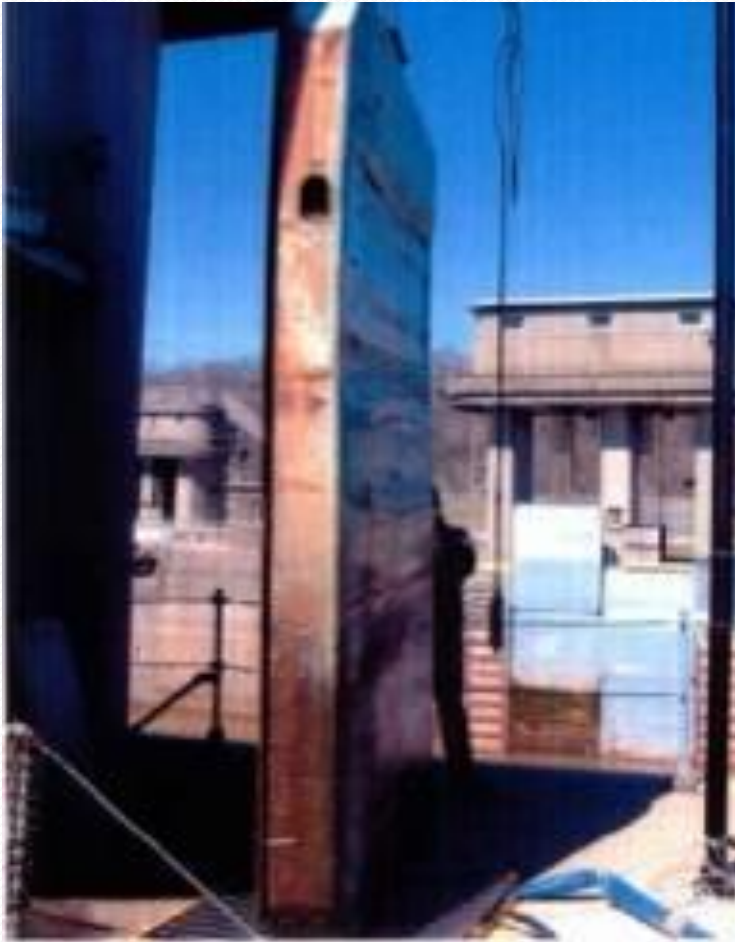
Current steel panels
