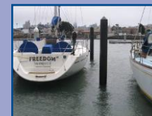
Pultruded piling in San Francisco
