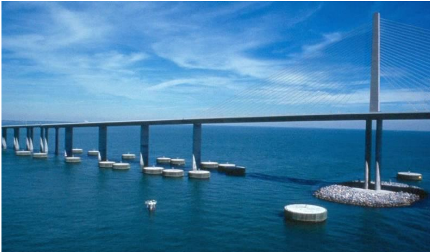
Sunshine Skyway Bridge
