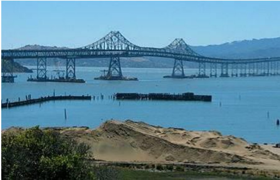
Richmond-San Rafael bridge (USA)
