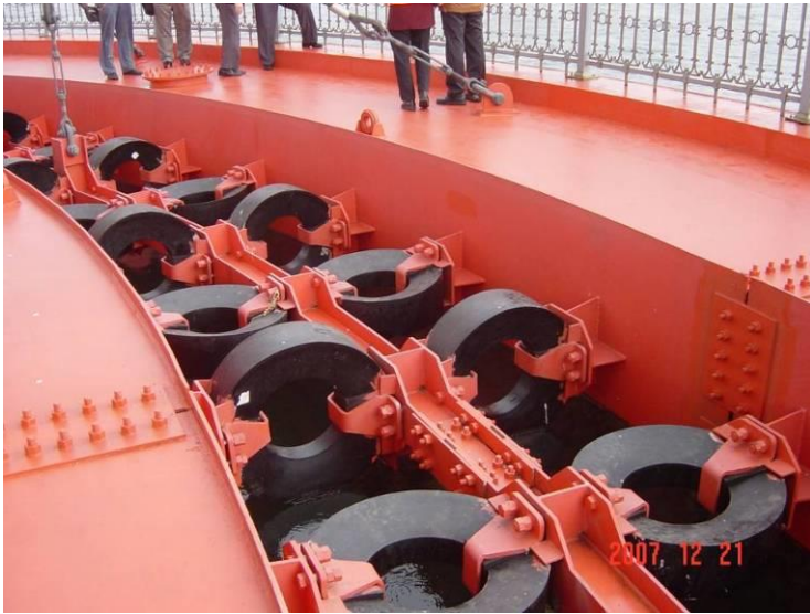
The Zhanjiang Bay Bridge
