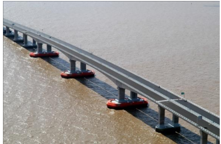
Pingtang bridge (old)
