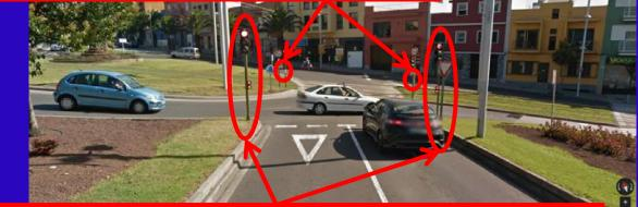
New traffic lights at the entrance to the roundabout that are close to the LRT tracks crossing
