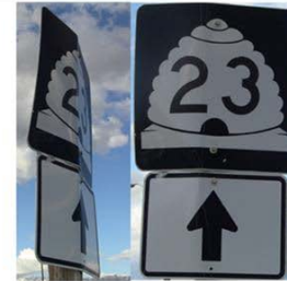
A. Bending Damage
