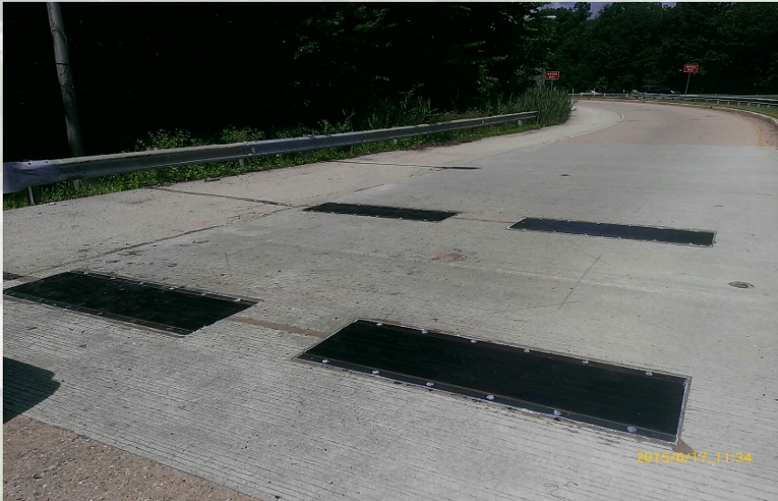
Ramp Rest Stop Bending Plates
