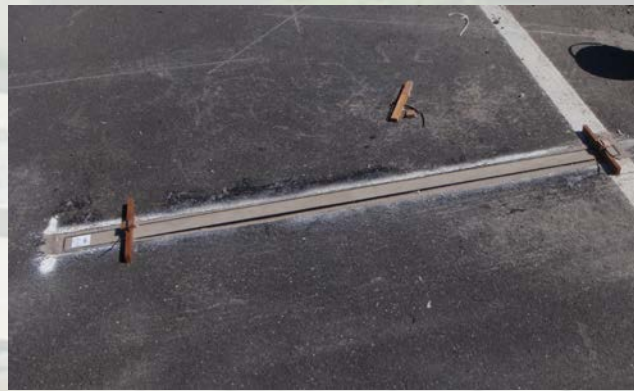
Newly Installed Mainline WIM Piezo
