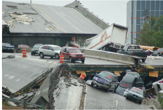
Problem Identification ( I-35W Collapse, Wikimedia )
