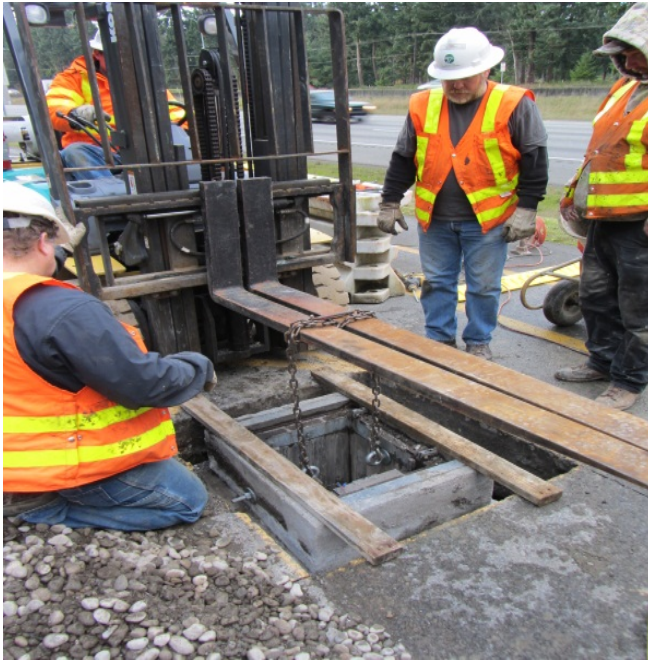
Installing camera jbox
