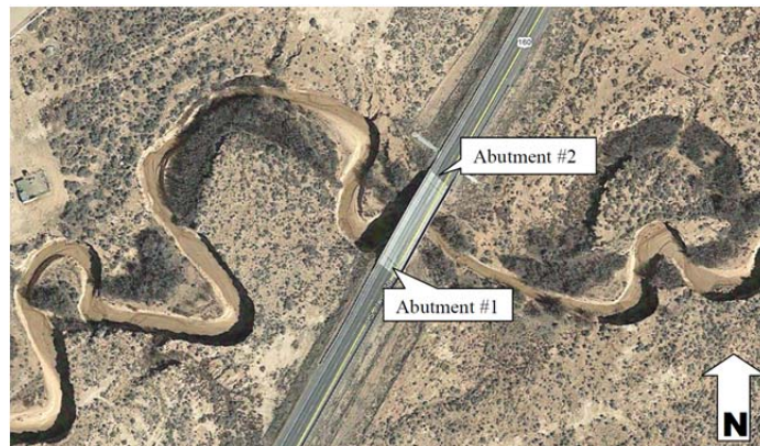
FIGURE 2 Aerial SR-160 Laguna Creek Bridge (Arizona DOT, 2016).
