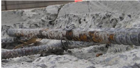
Rebar Corrosion
