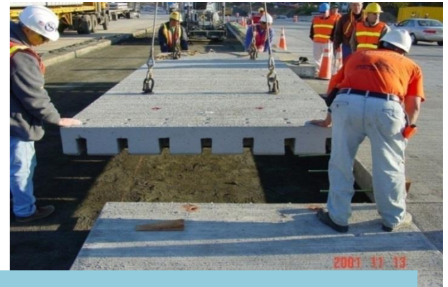
Conventional Jointed PCP System – top or bottom dowel slots
