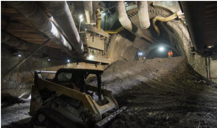
Chinatown Station Construction
