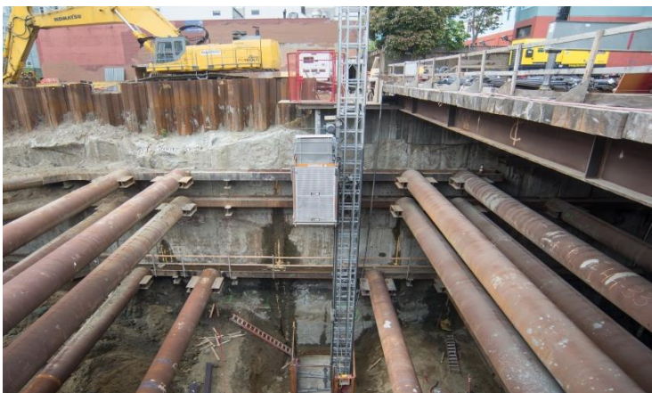
Moscone Station Construction
