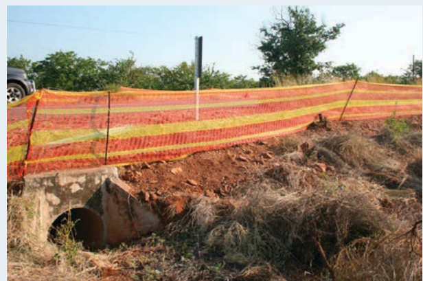
Under-road culvert with drift fencing
