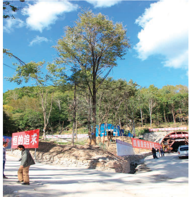
Figure 4. Retaining Wall for Vegetation
