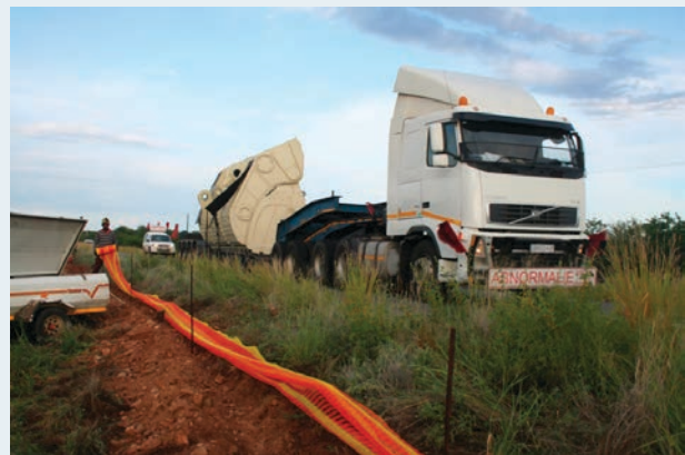
Assembling the fence
