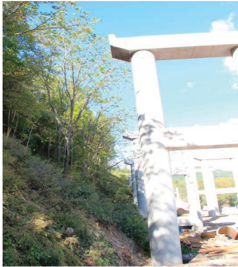
Figure 6. Vegetation Conservation Near Bridge Construction
