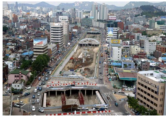
June 2004 Under Restoration
