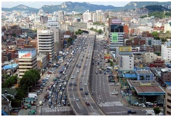
June 2003 Before Restoration
