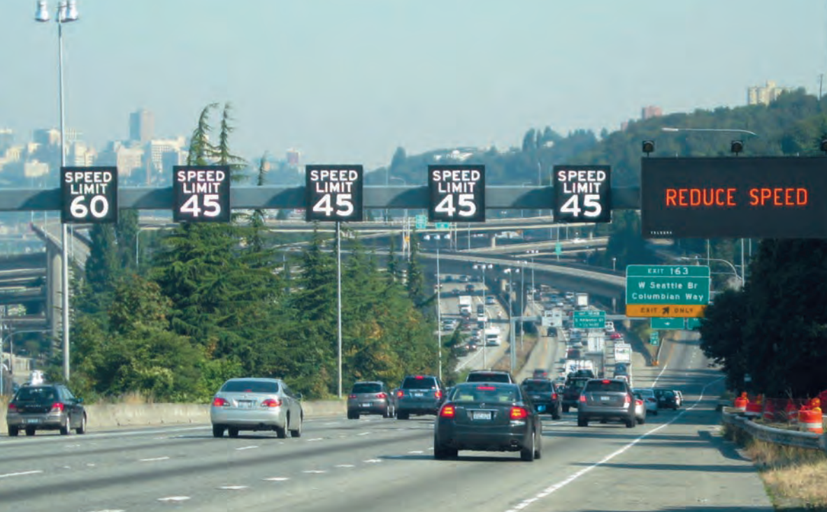
Dynamic message signs alert motorists to upcoming congestion. On many of the nation's highways, population and traffic growth have outstripped capacity.
