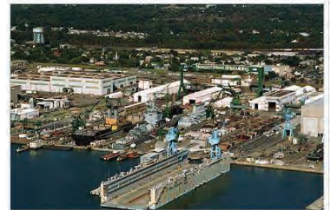
Aerial view of the Newport News shipyard
