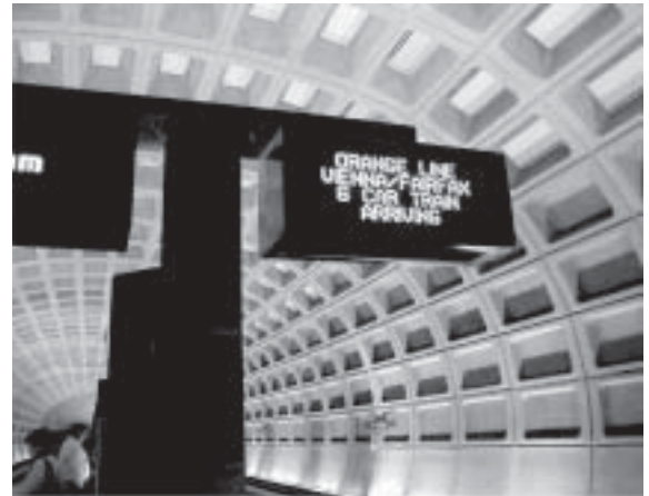
A real-time passenger information display system in the Washington, D.C., Metro, detailed in TCRP Report 92, Strategies for Improved Traveler Information , provides actual arrival times of trains, elevator and escalator outages, incident information, and security alerts.
