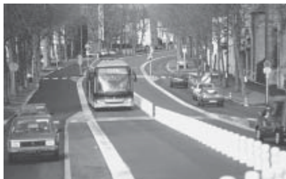
Bus rapid transit vehicles, the subject of TCRP Report 90, Volume 1, Bus Rapid Transit: Case Studies in Bus Rapid Transit , operate primarily in fast and easily identifiable exclusive transitways or dedicated bus lanes.
