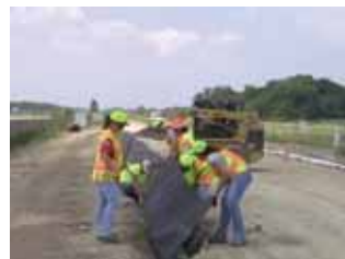
Tying G CBD into edgedrain during installation in a Minnesota DOT test track (left), and covering the G CBD with base course aggregate in the test section (right).
