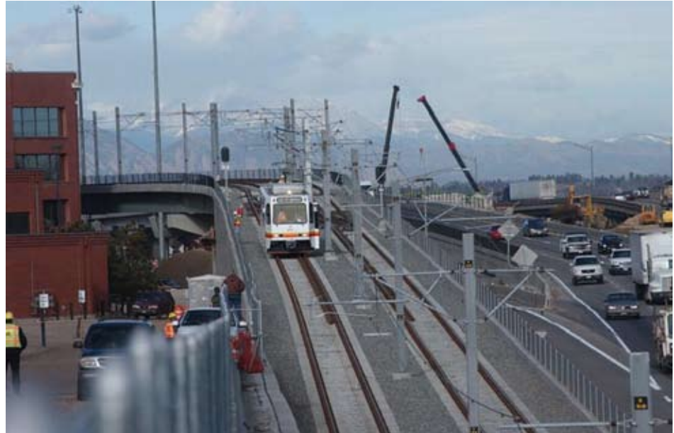
Light rail junction at interchange of I-25 and I-225 in Denver. (Photo courtesy of Richard F. Clarke.)
