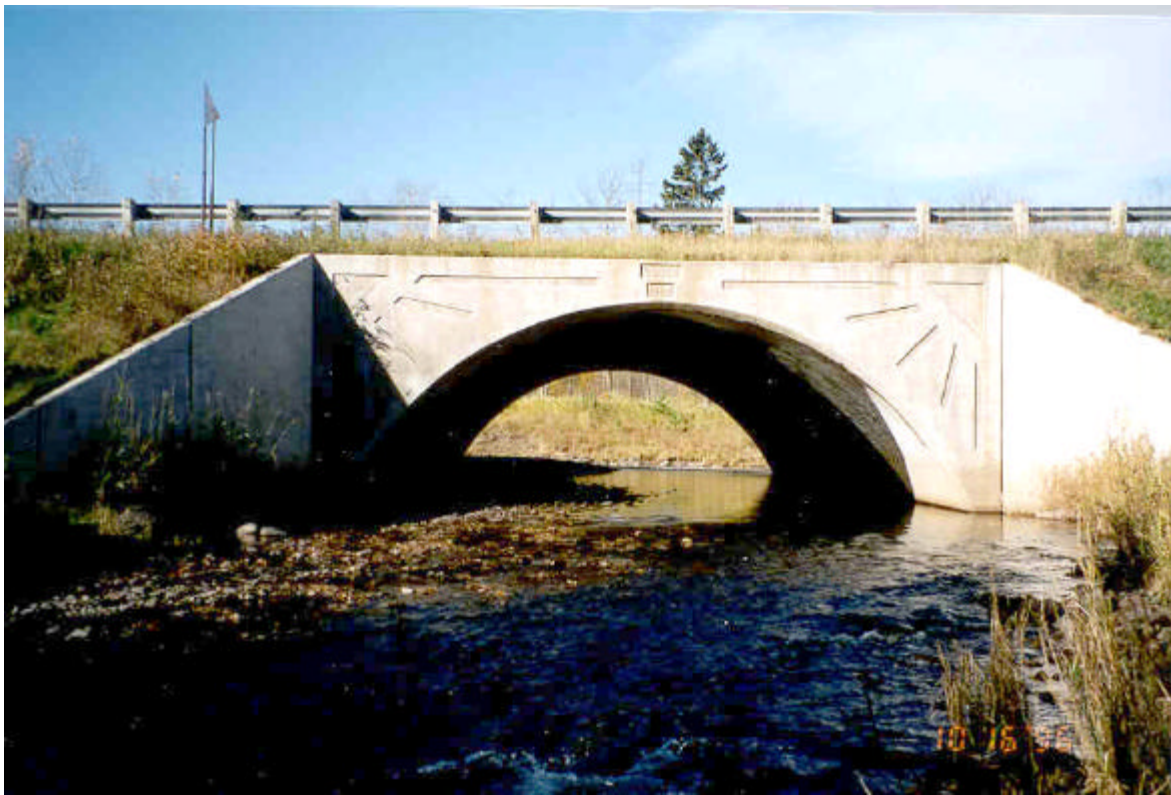
FIGURE 3 Typical long-span culvert (44-foot span).
