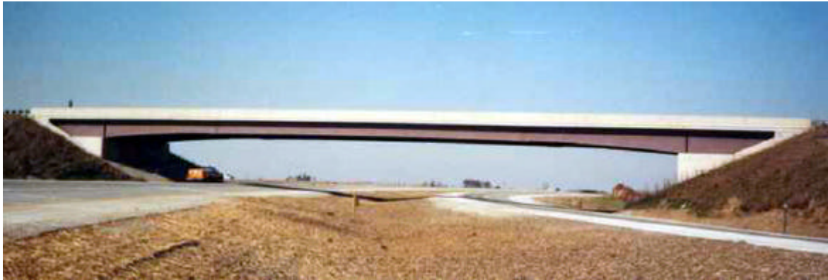
FIGURE 2 Steel bridge clear-spanning an entire freeway.
