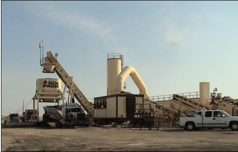
Figure 29 Portable Asphalt Plant used for Graham, TX Project
