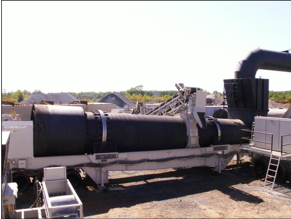
Figure 18 Portable Asphalt Plant used for Iron Mountain, MI Project (19)
