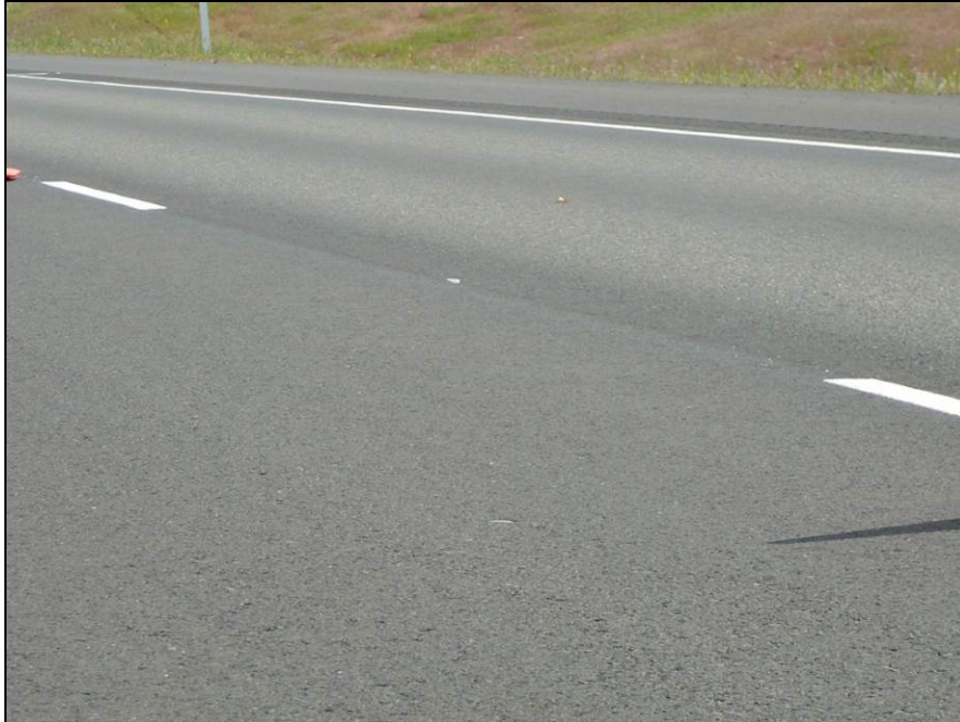
Figure 47 WMA (Foreground) and HMA (Background) Sections at 13-Month Inspection to Walla Walla, WA
