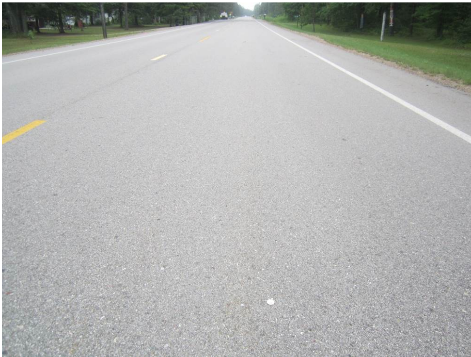
Figure 66 HMA Control Section at 22-Month Inspection in Rapid River, MI
