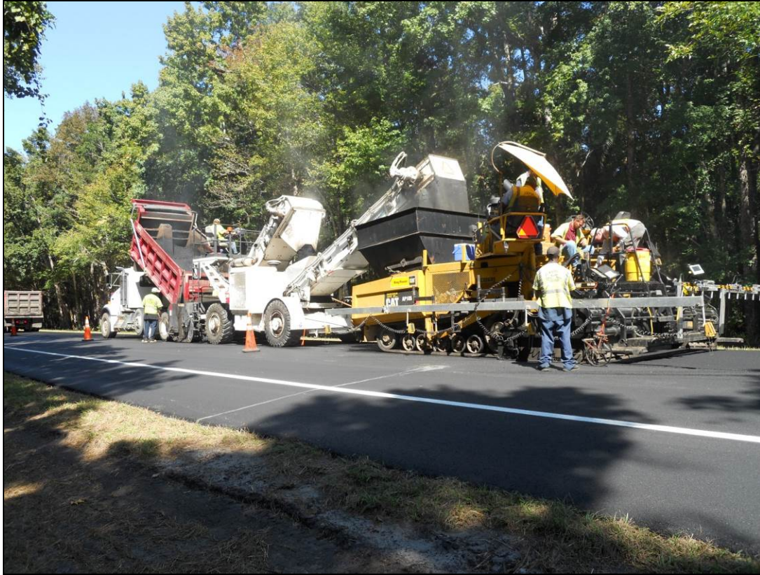
Figure 96 MTV Transferring Mix into the Paver in Jefferson County, Florida
