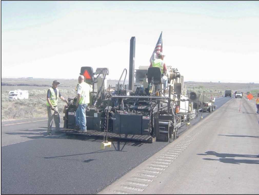
Figure 37 Paver Spreading Mix in George, WA
