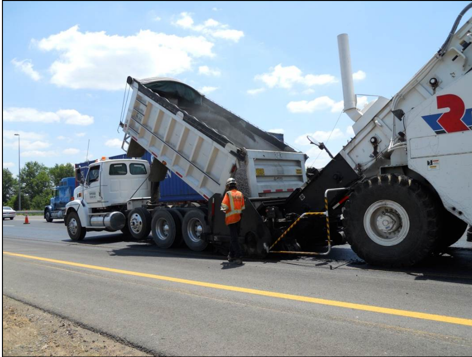
Figure 55 Truck Dumping into MTV in Centreville, VA
