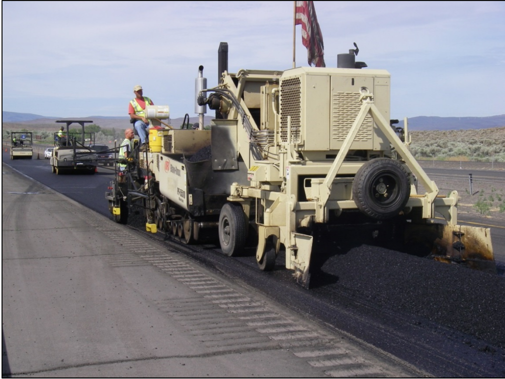
Figure 36 Windrow Elevator Transferring Mix to Paver in George, WA
