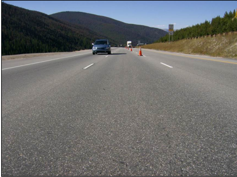
Figure 24 Surface Texture of Test Sections in Silverthorne, CO
