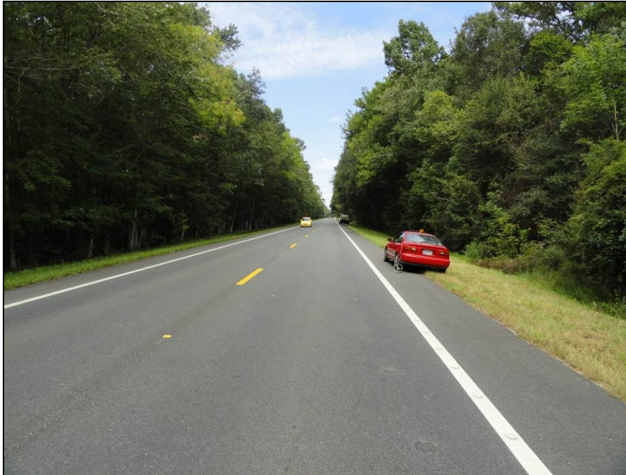
Figure 97 WMA (left lane) and HMA Control Sections (right lane) in Jefferson Co., FL
