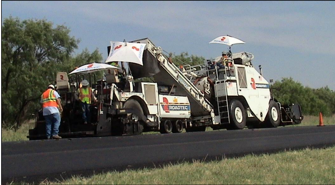
Figure 32 Material Transfer Device and Paver used for Graham, TX Project
