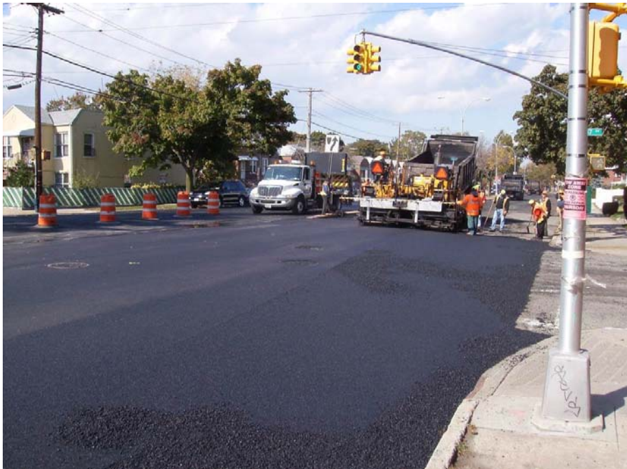
Figure 112 Typical Handwork in Urban Paving Project
