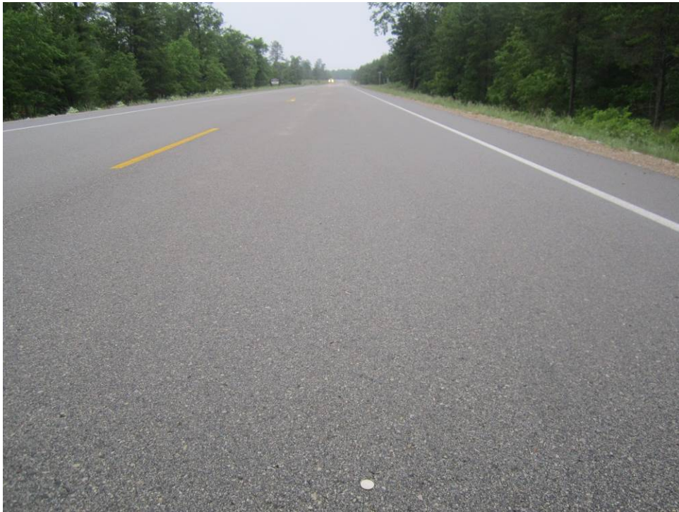
Figure 68 Evotherm 3G Section at 22-Month Inspection in Rapid River, MI
