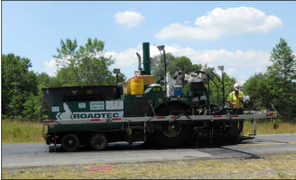
Figure 57 RoadTec RP-190 Paver used in Centreville, VA
