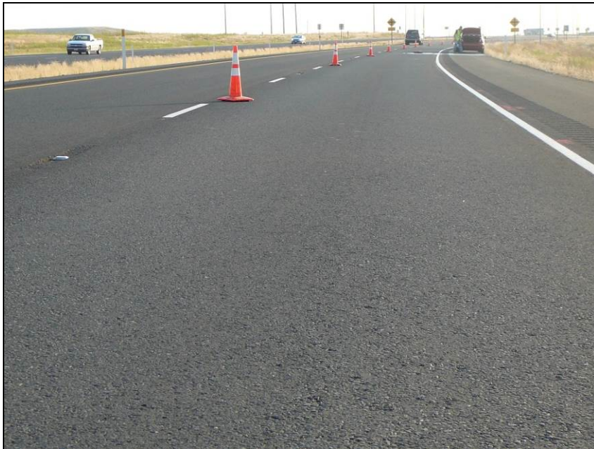
Figure 50 Example of Surface Texture at 27-Month Inspection in Walla Walla, WA
