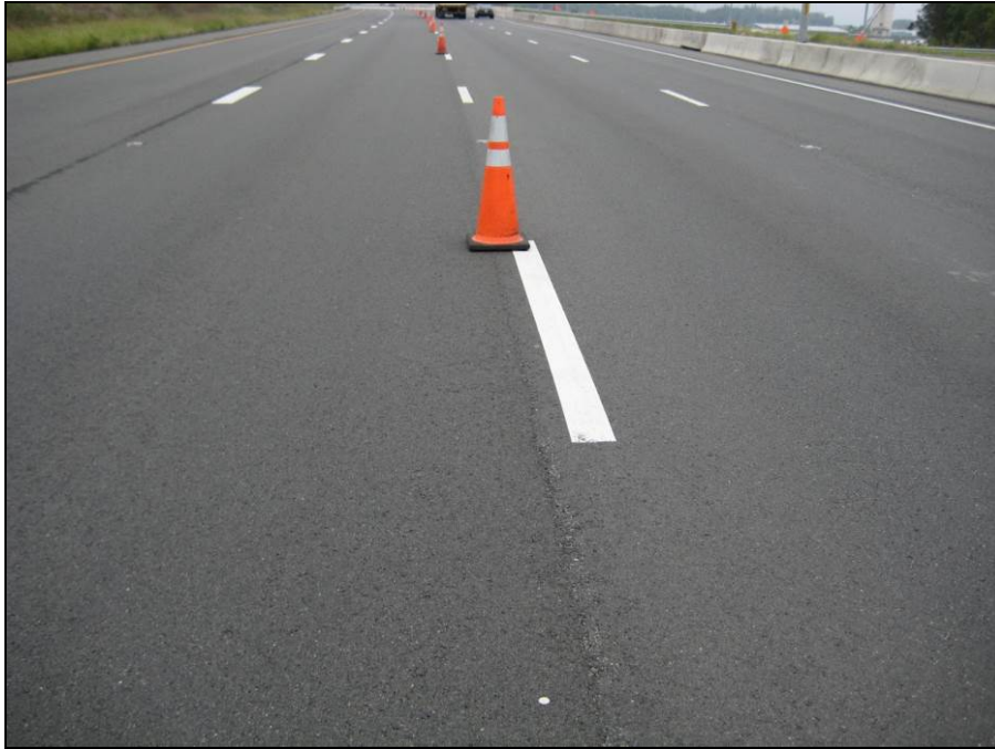
Figure 59 WMA and HMA Sections at 15-Month Inspection in Centreville, VA
