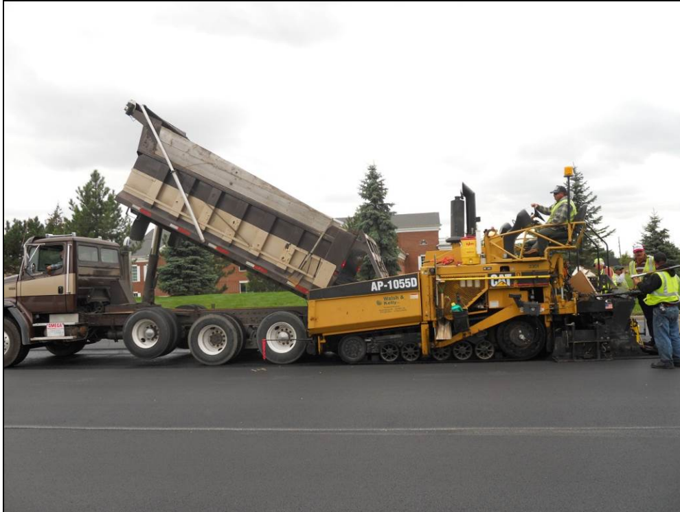
Figure 85 Truck Dumping into Caterpillar AP-1055D Paver
