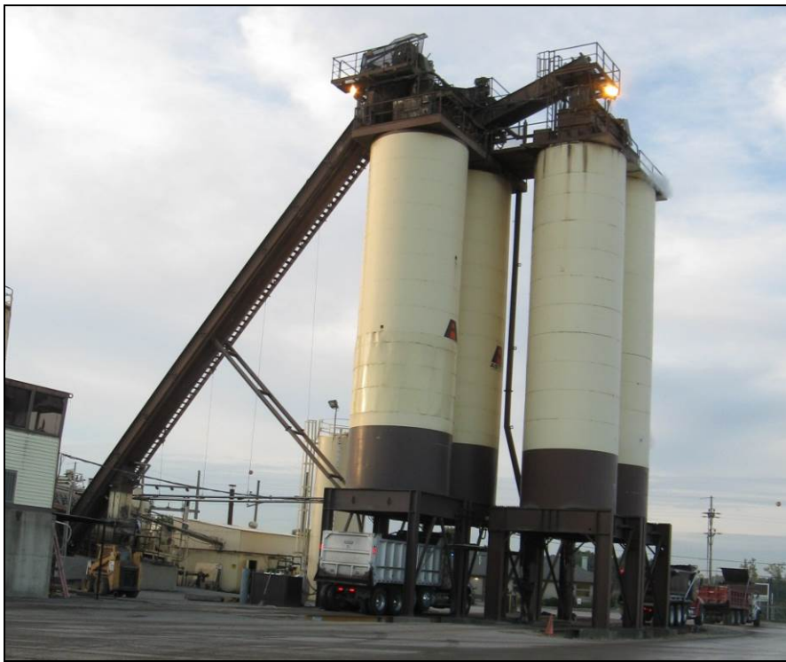
Figure 83 Counter-Flow Drum Plant in Griffith, IN
