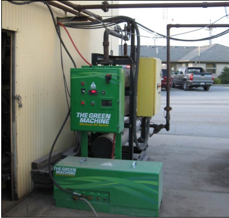
Figure 82 Ultrafoam GX2 Foaming System used in Munster, IN
