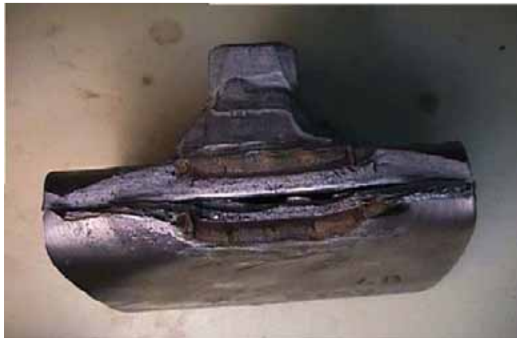
Figure 2.2. Fatigue Crack at End of Horizontal Gusset Plate Connection. Cook et al. (2000)
