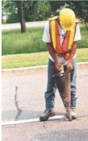
Photograph 4-13: Application of Emulsion Crack Treatment (24)
