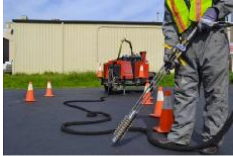
Photograph 4-9: Hot Air Lances (Courtesy Crafc0, Inc.) (Courtesy Lab Mfg.)
