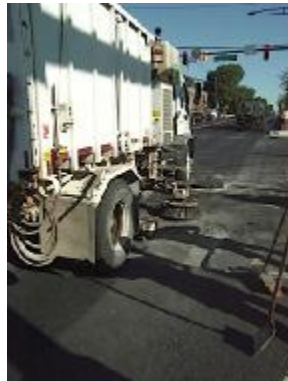
Photograph 4-6: Pavement Sweeping (Photograph by Dale Decker)
