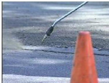
Photograph 4-7: Compressed Air cleaning of crack (Courtesy Crafcoc)
