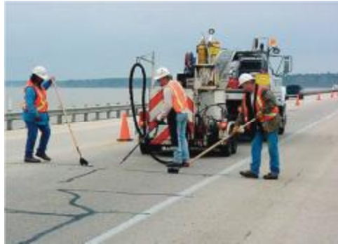
Photograph 4-15: Crack Treatment Operations (21)
