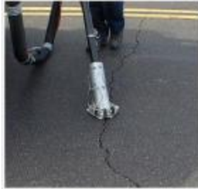
Photograph 4-8: Crack Vacuum (Courtesy Crafcoc)
