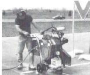
Photographs 4-4: Diamond Saw Crack Cutting (16)
