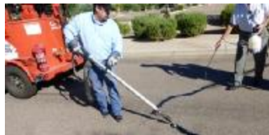
Photographs 4-14: Blotter Applications ((A) Sand Blotter and (B) Toilet Paper from (16)), ((C) Anti-Tracking Solution by Dale Decker)
