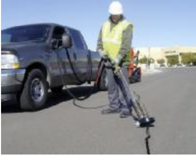
Photograph 4-9: Hot Air Lances (Courtesy Crafc0, Inc.) (Courtesy Lab Mfg.)
