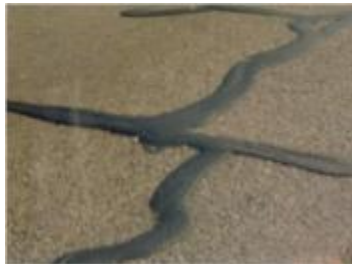
Photograph 4-3: Excessive Overbanding (22)
