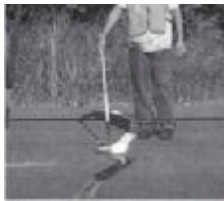
Photographs 4-14: Blotter Applications ((A) Sand Blotter and (B) Toilet Paper from (16)), ((C) Anti-Tracking Solution by Dale Decker)
