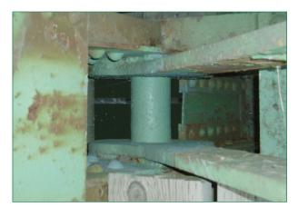
Figure 3-2 Pack rust between eyebar head and adjacent gusset plate before ultra-high-pressure washing
