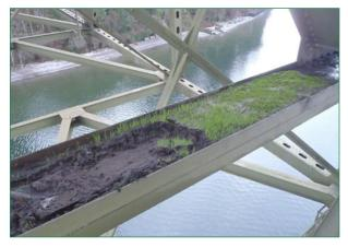
Figure 3-4 WSDOT bridge before cleaning
