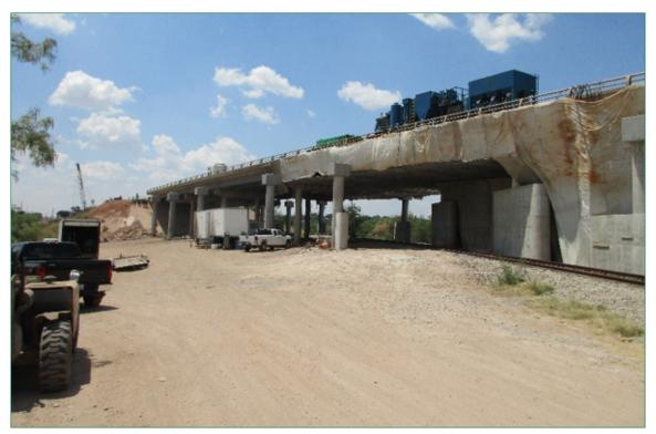
Figure 2-2 Containment for US 67 over Texas Pacifico Railroad in Ballinger, TX
