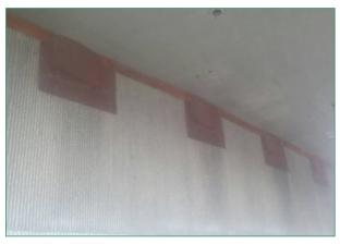
Figure 3-5 Screening used on WSDOT bridges to keep birds out
