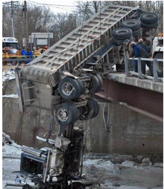
Figure 5. Tractor trailer truck penetration of bridge rail, Glenmont, NY.
