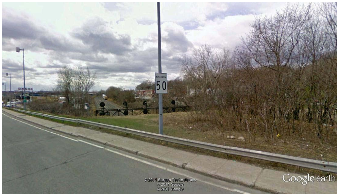
Figure 14. W-beam Guardrail Roadside Barrier, Montreal, Quebec. [Google Earth]
