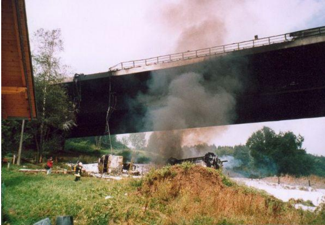
Figure 6. Tractor trailer truck which penetrated the Wiehlthal Bridge, Germany. [Wiehlta04]
