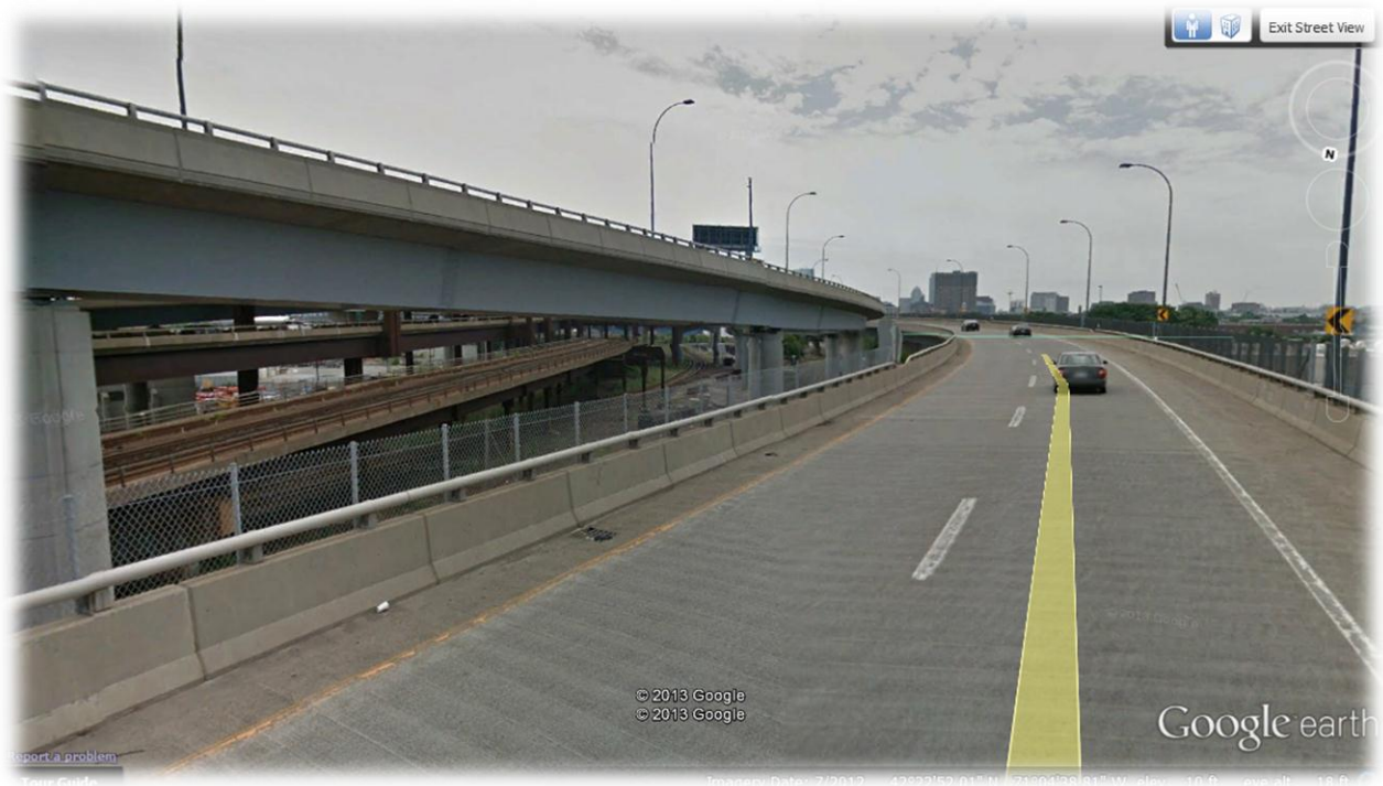
Figure 22. Close-Up of Bridge Rail Type (upper left) and Exit 26 Ramp Truck, Boston, MA. [Google Earth]
