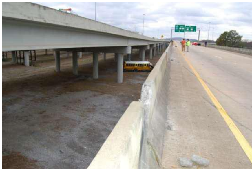
Figure 29. Final rest position of a school bus that penetrated a concrete bridge railing near Huntsville, AL in 2006. [NTSB09b]
