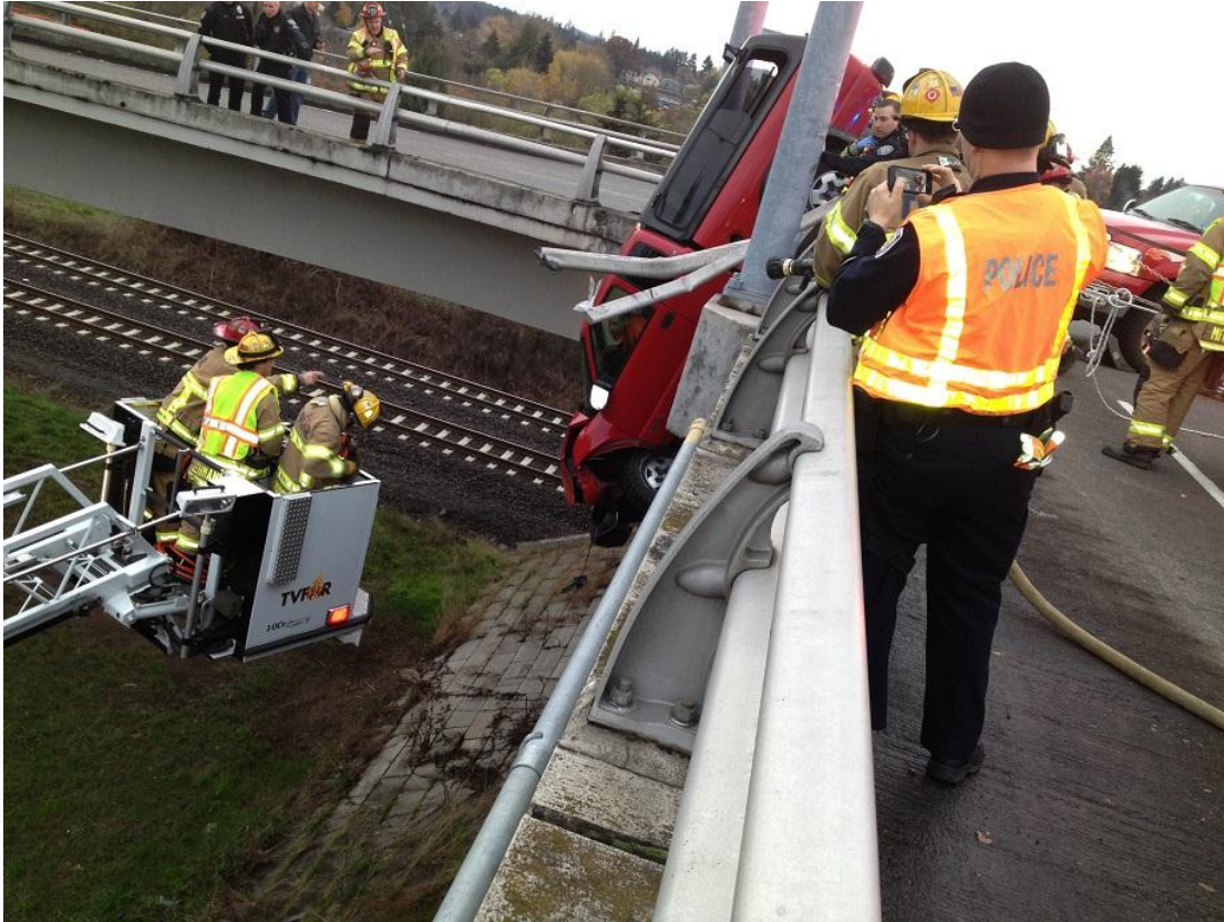
Figure 16. Pickup Truck After Rail Penetration, Beaverton, OR. [ORHER01]
