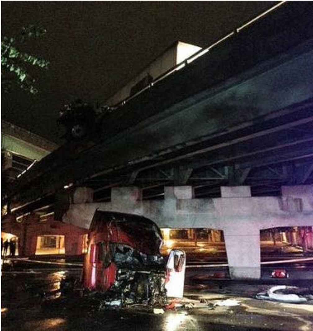
Figure 11. Cab of tractor-trailer penetrated rail and fell to road below, trailer remained on bridge, Syracuse, NY. [Syracuse12]
